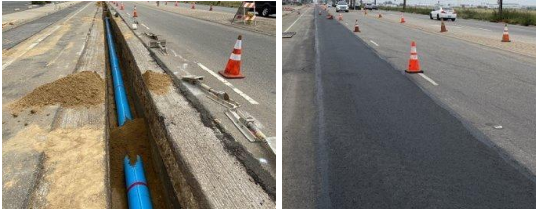
Figure 1 – Utility Trench and Trench Patch
