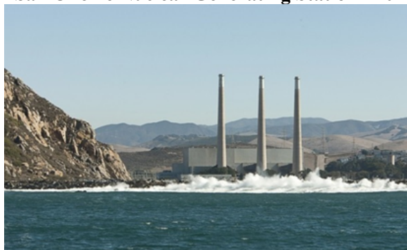
Morro Bay Power Plant - 2014
