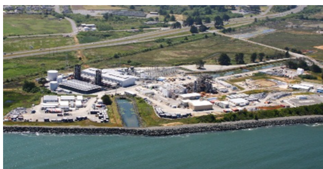
Humboldt Bay Power Plant - 2010
