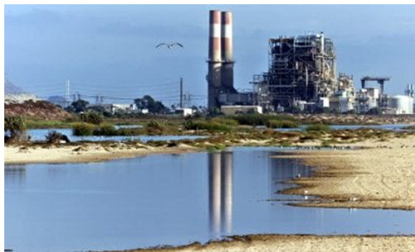
Mandalay Power Plant: 1956 - 2018
