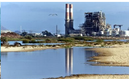
Mandalay Power Plant - 2018
