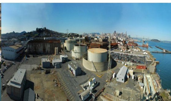
Potrero Generating Station - 2011
