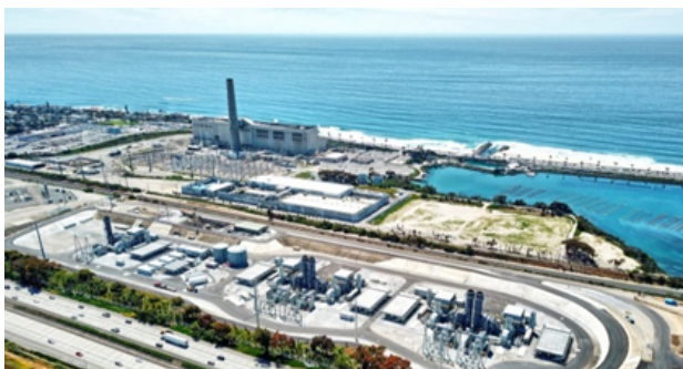
Encina Power Plant - 2017
