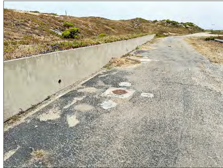
Photograph 2: Overview of MW-5A, looking northeast (7/18/2024).
