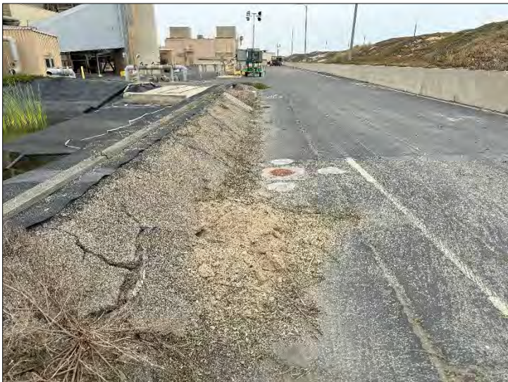
Photograph 3: Overview of MW-10, looking northeast (7/18/2024).
