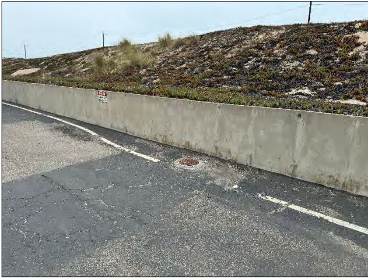
Photograph 5: Overview of MW-36, looking south (7/18/2024).
