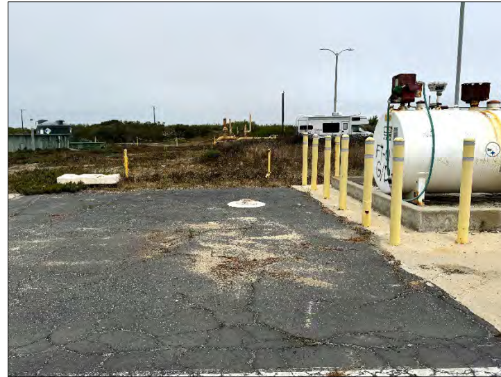
Photograph 10: Overview of well MW-44, looking north (7/18/2024).
