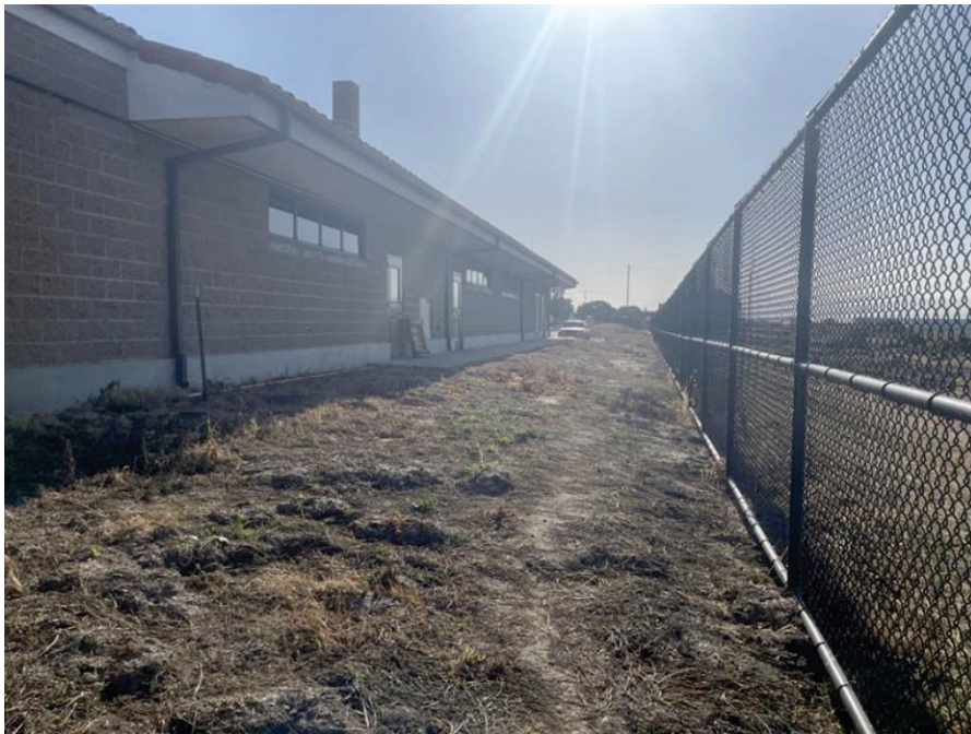
Photo 6: View looking east along southern project boundary.
