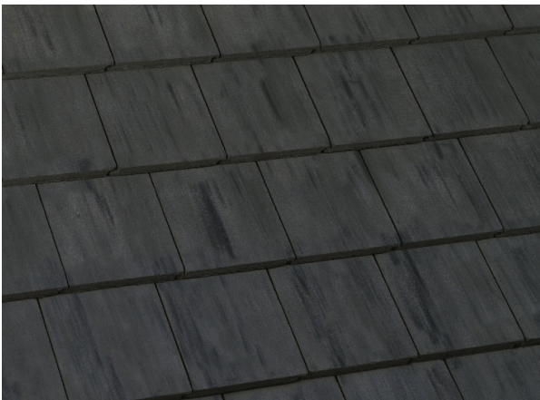
RT#1 ROOF - LIGHTWEIGHT CONCRETE TILES MATCH EXISTING BUILDING B
