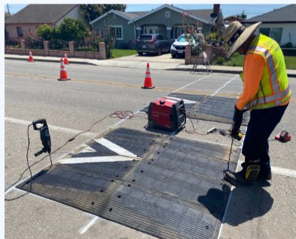
Speedhumps Installation
