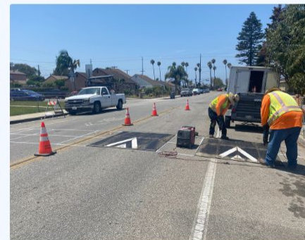
Speedhumps Installation
