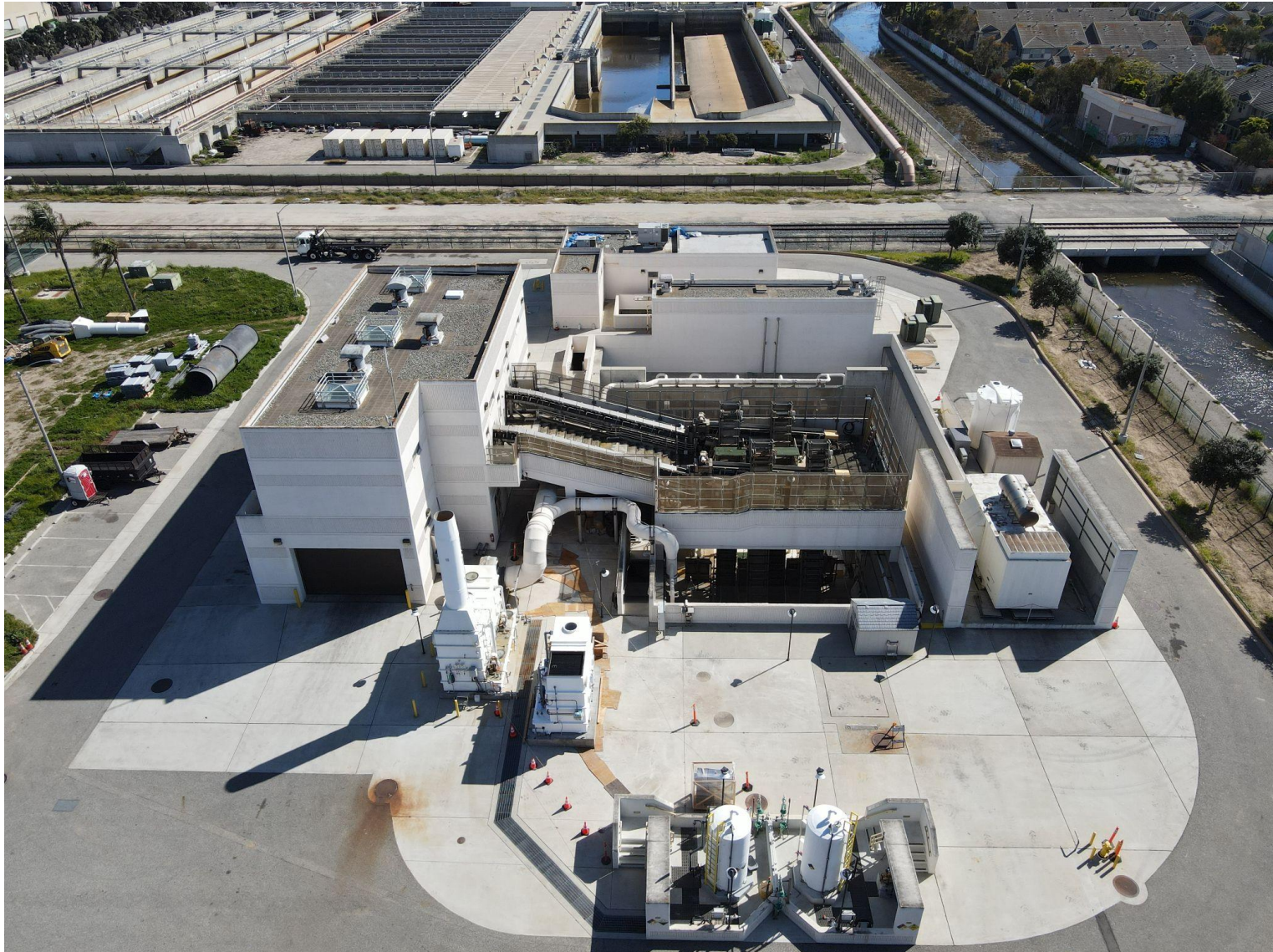
Wastewater Headworks Facility - 5741 Perkins Rd
