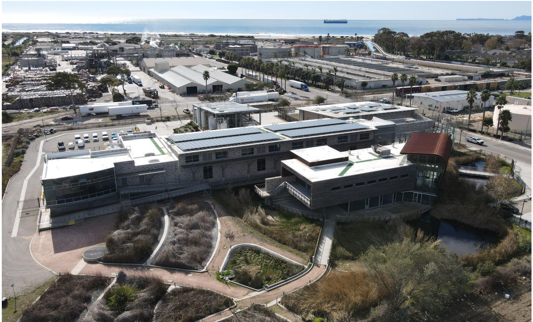
Advanced Water Purification Facility - Water Division
