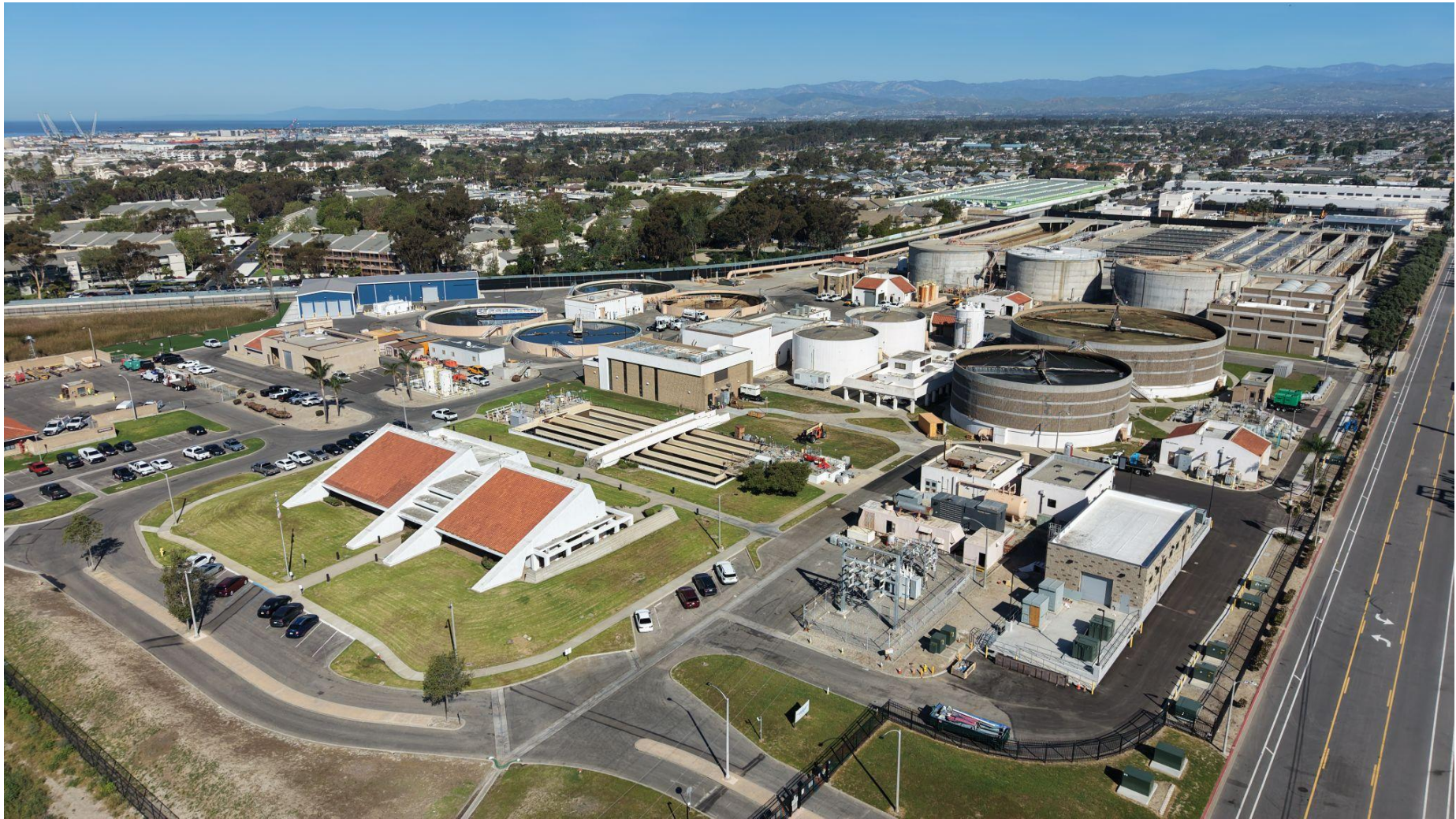
Water Resource Recovery Facility - Wastewater Division
