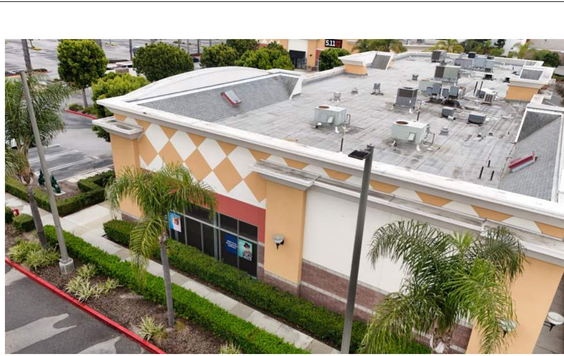
EXISTING LED SITE LIGHT - C
