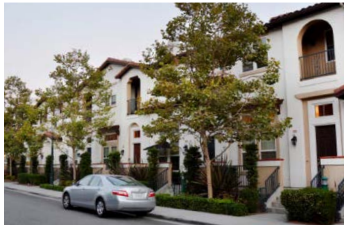
A raised and set back ground floor provides privacy to residences.
