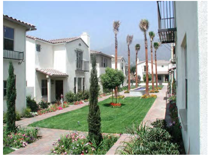
This paseo is a good example of an extensions of the public realm. It leads the pedestrian from the sidewalk, into the site where individual units are accessed.
