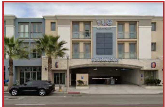
DON'T: The parking entrance dominates the composition, interrupting the ground floor frontage. Its width, height, central location, and even signage make the entrance more conspicuous than it needs to be.
