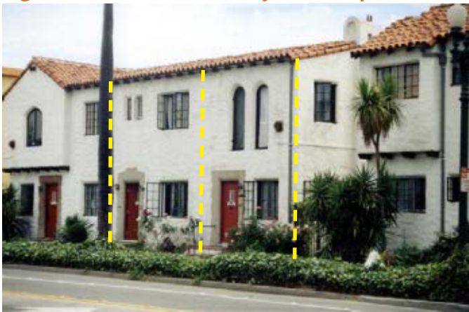
Upper floor windows are grouped and stacked above ground floor openings to create coherent compositions which correspond to the dwelling units within. Divisions between units are noted above with yellow dashed lines.
