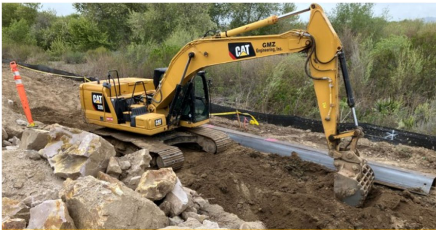
Santa Clara River Levee (SCR-3) Ph 2
