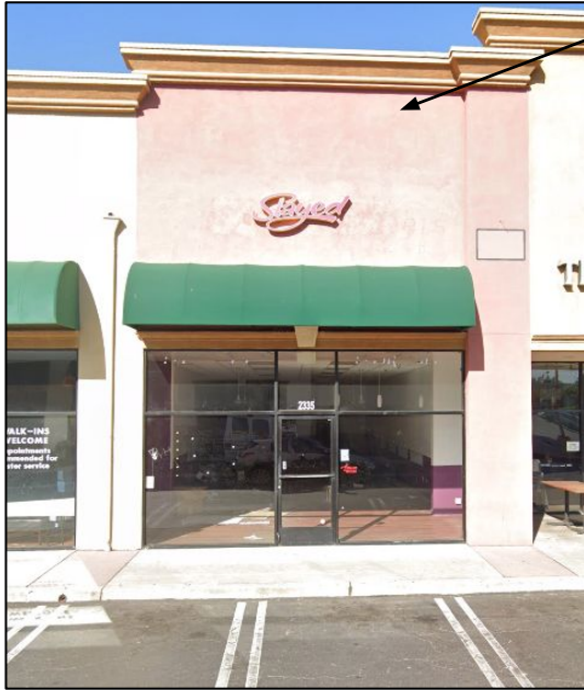
View from parking lot, looking west
