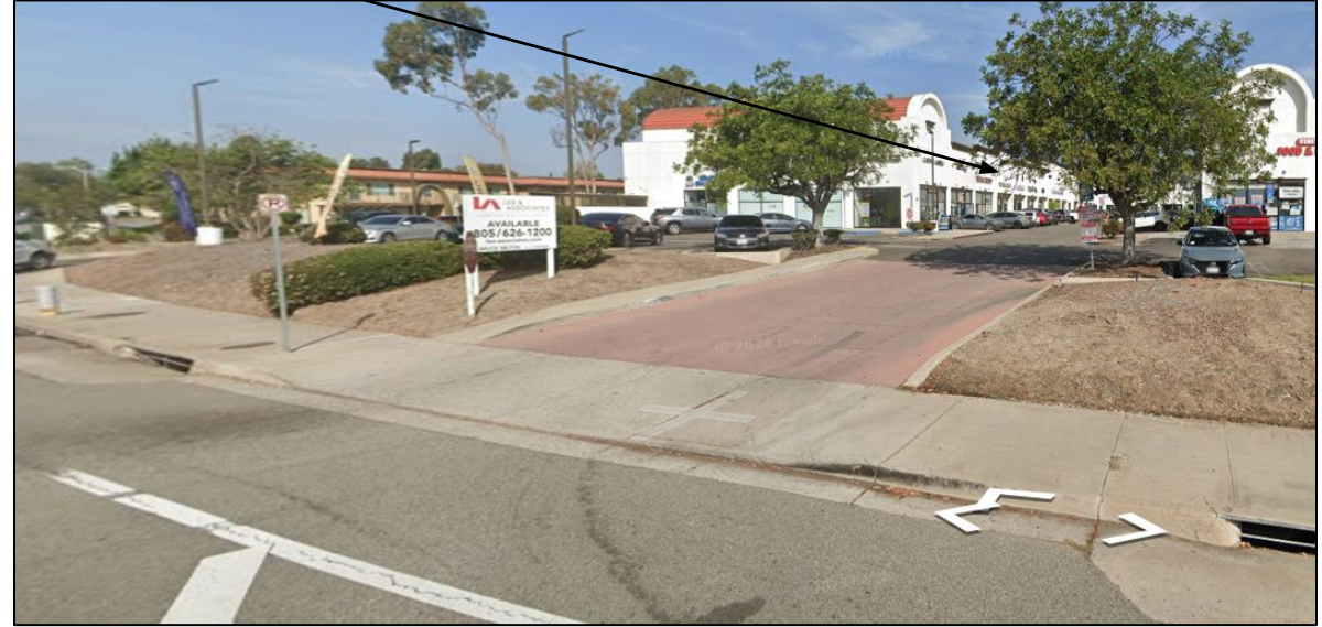
View from West Vineyard Avenue, looking northwest
