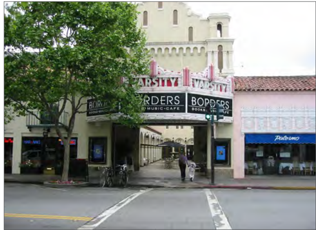
Example of a covered passage.
