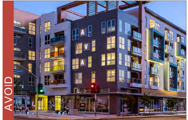
Example of facades articulated through the use of applied frames, currently in fashion but likely to look dated before long.
