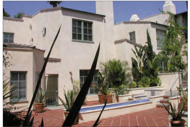
Plaster walls with pre-cast concrete caps.
