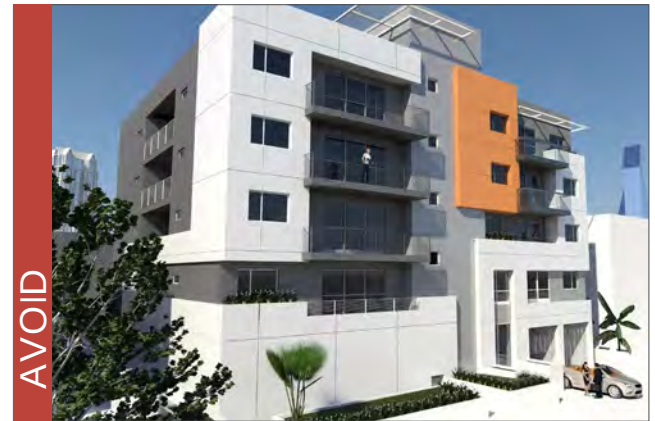
A blank ground floor frontage.
