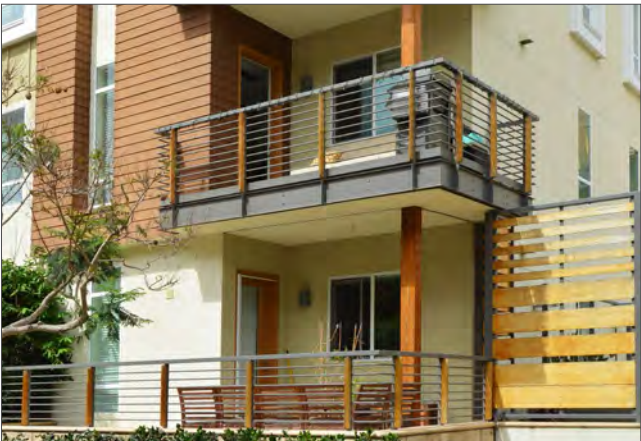
A wood balcony supported by extended beams.
