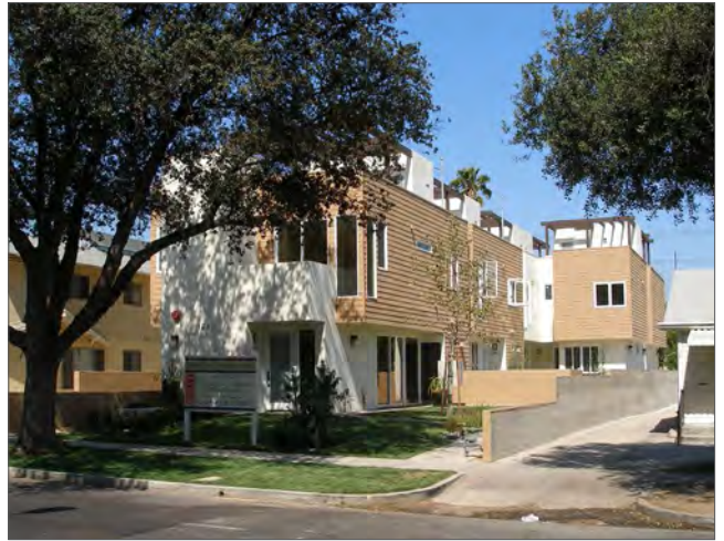
Multiple roof decks on one building.
