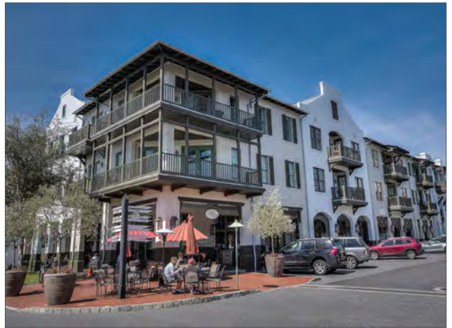
Corner balconies above a cafe.
