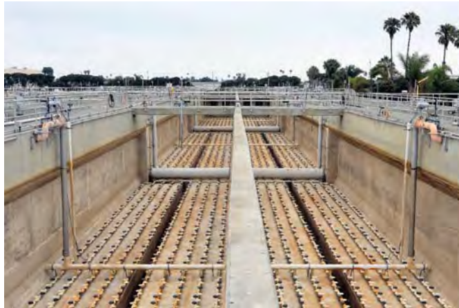
Activated Sludge Tank
