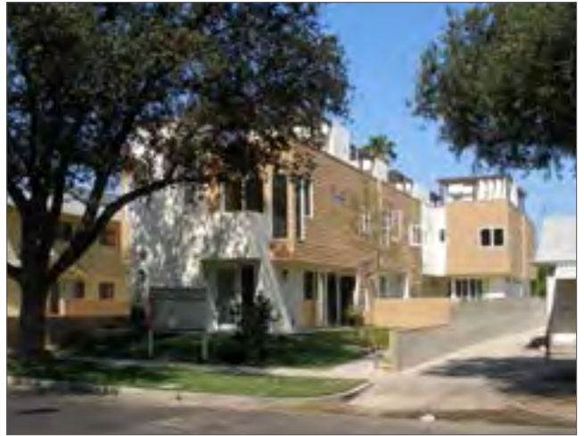
Multiple roof decks on one building.
