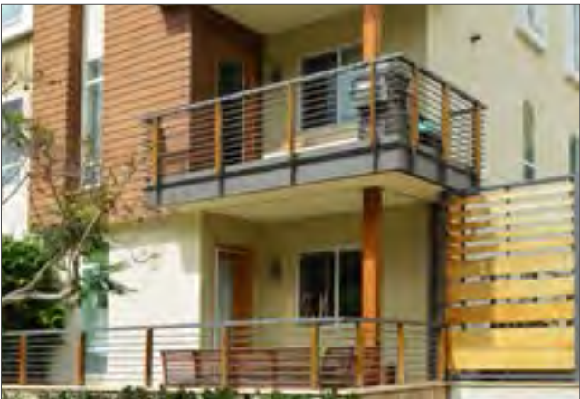
A wood balcony supported by extended beams.
