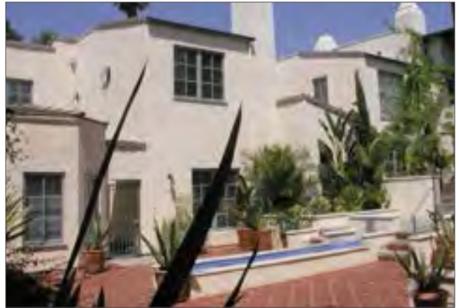
Plaster walls with pre-cast concrete caps.
