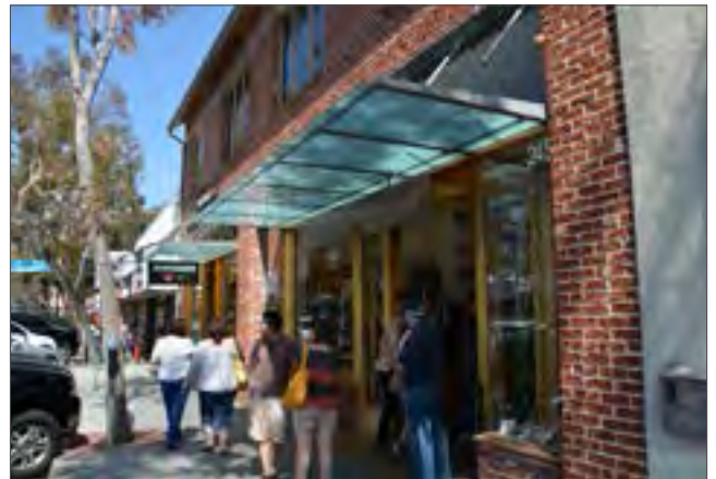
A glass awning demarcating a store entrance.
