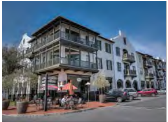
Corner balconies above a cafe.
