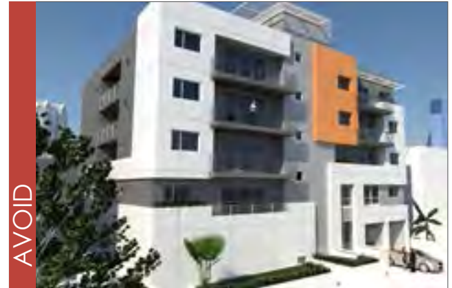
A blank ground floor frontage.
