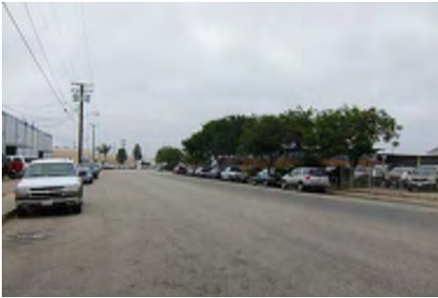
Commercial Avenue is extremely wide with no defined lanes.
