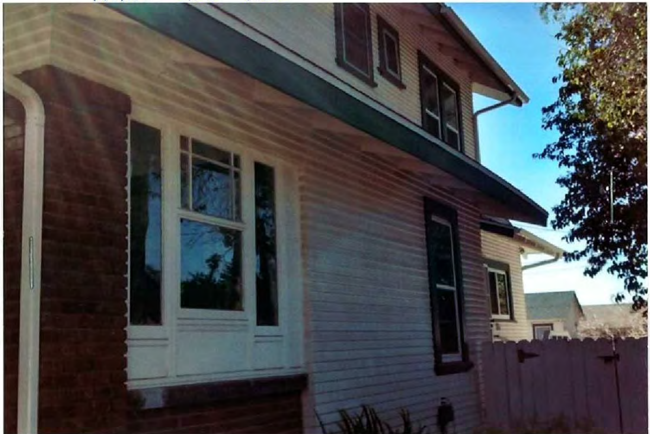
NORTH SIDE VIEW
