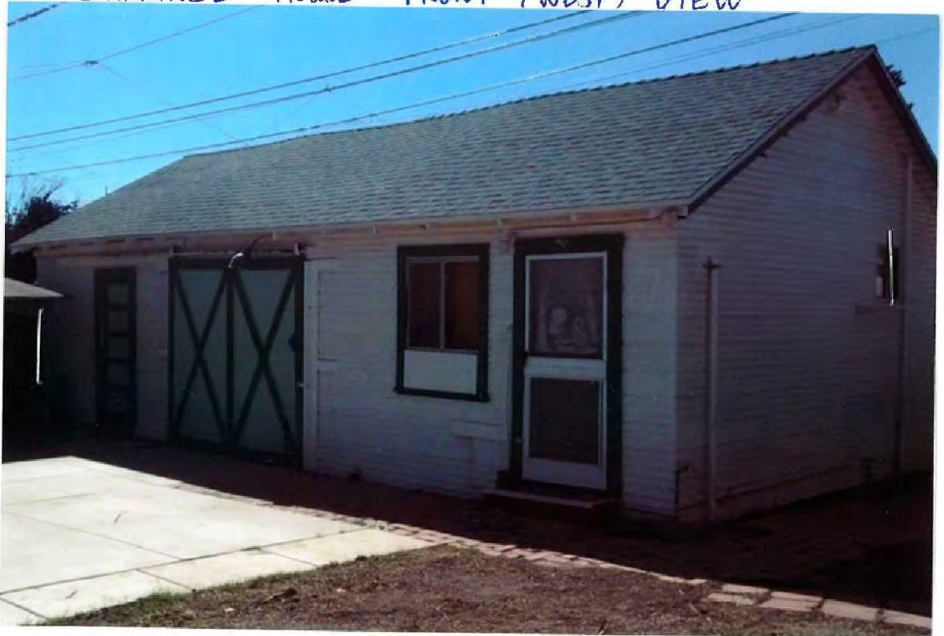
CARRIAGE HOUSE FRONT (WEST) VIEW
