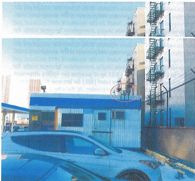
Fig. 1. The three vent pipes (enclosed by the red ellipse) on the right side of the convenience store of a gas station are <10 m away from the residential building. (For interpretation of the references to color in this figure legend, the reader is referred to the web version of this article.)
