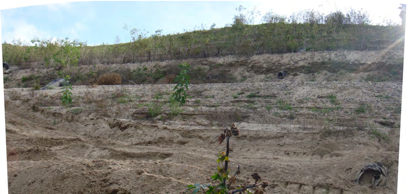
Photo #13. East corner slope area. Note cut off drains in slope face.
