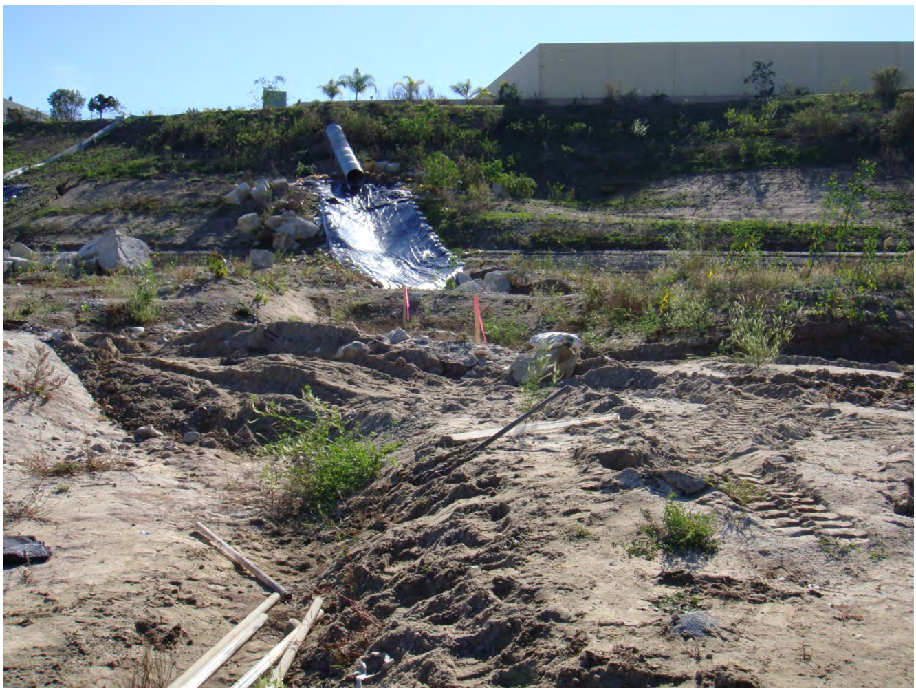
Photo #4. Area# 1, looking Southeast across fan. Stormdrain and two boring locations shown in center.
