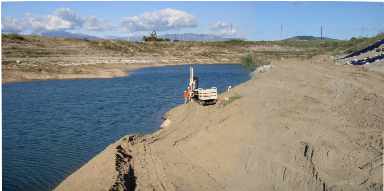
Photo #6. Area #2, looking North showing access ramp and rig set up on boring S12, stormdrains to right.
