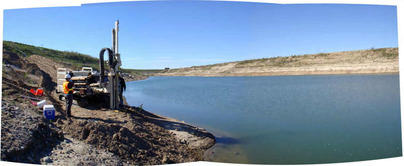
Photo #10. Looking Southwest across Area #3 showing sediment fan and rig set up on boring.
