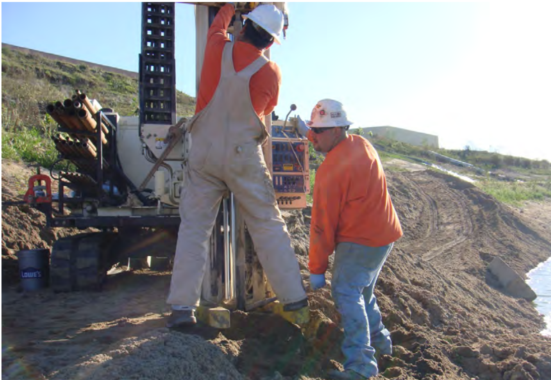
Photo #8. Area #2, looking South with rig set up on sediment fan at boring location S10.
