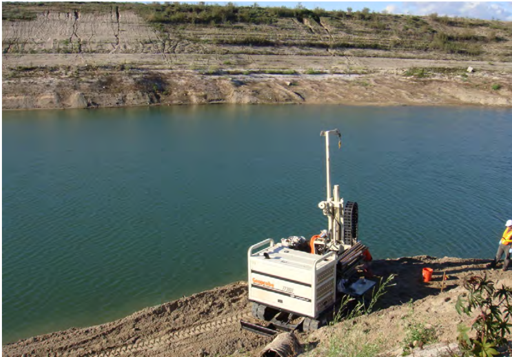
Photo #7. Area #2 looking Northwest, showing rig set up at water's edge on fan.
