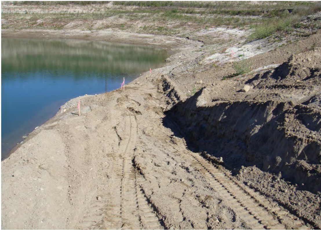
Photo #9. Access cut down to Area #3. Note stakes at boring locations.
