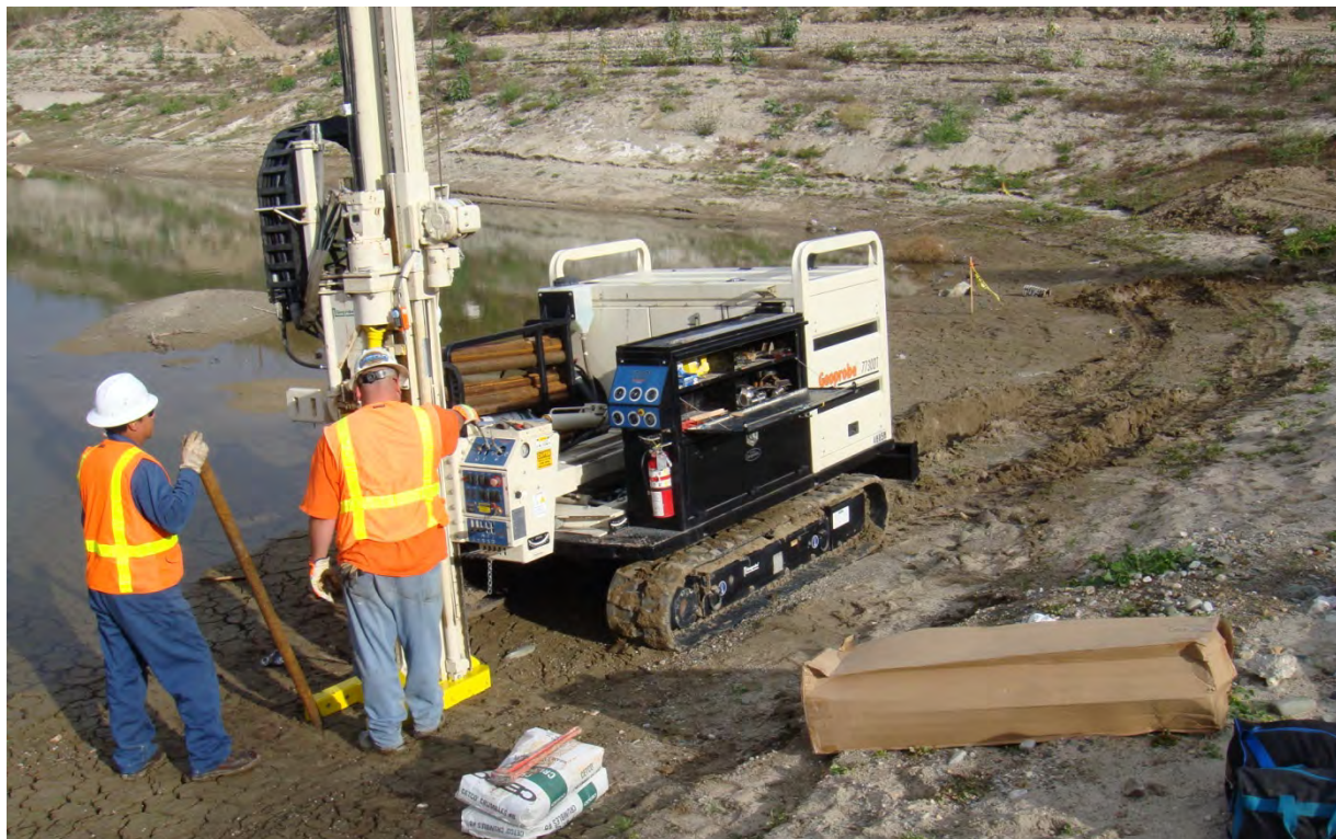
Photo #14. Area #4, rig set up on boring S2 at water's edge.
