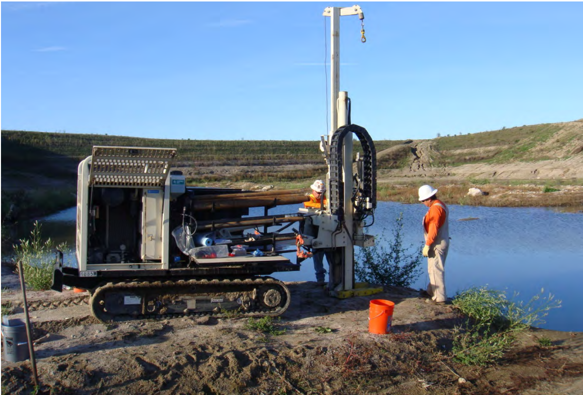
Photo #5. Area #1 showing Geoprobe rig set up on boring S5.
