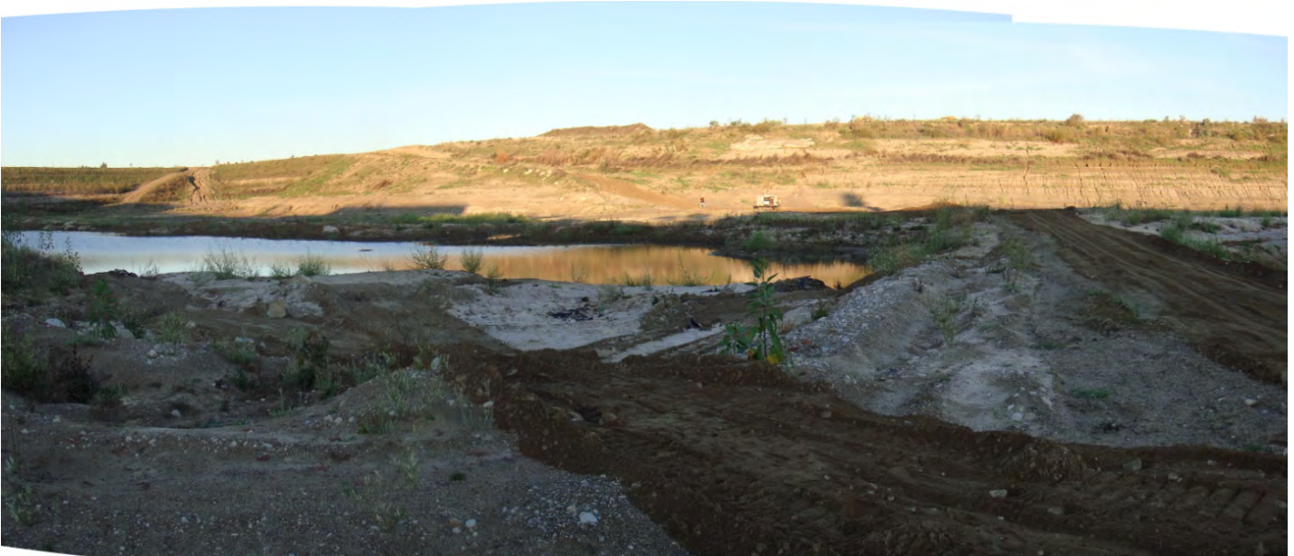
Photo 1. Panoramic view of Area #1 looking Northwest, sediment fan visible left of road.
