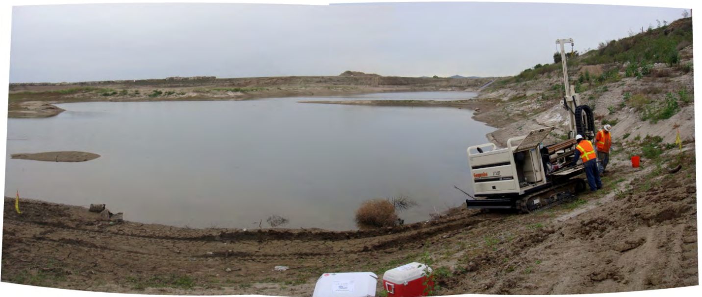
Photo #12. Looking Northwest from Southeast corner of pit. Rig set up at Area #4 sediment fan.
