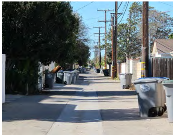
Top - Figure 3.27 Asphalt Alley in Oxnard
