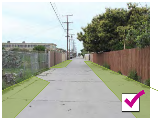
Figure 6.09 Paving & Traffic Patterns Site Criteria Top: Poor paving in an Oxnard alley; Center: Poor traffic patterns for Green Alley design; Bottom: Favorable traffic patterns for Green Alley Design.
