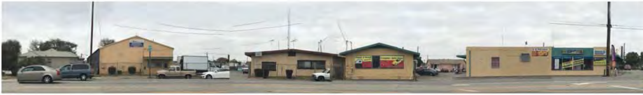
11 SITE ADJACANT- WEST VINEYARD AVE. - NORTH OF SITE
