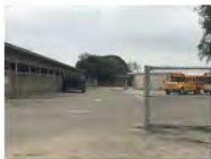
5 EXISTING SITE - E. VINEYARD AVE. INSIDE THE SITE
