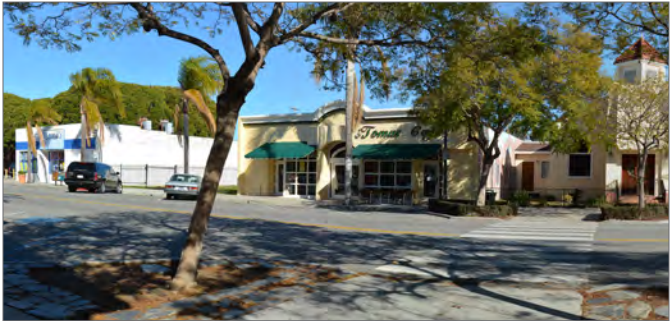
Existing Condition: The landscape of A Street is minimal and not well maintained. The mid-block jacaranda trees are lovely, but the ground plants could be very easily improved. The queen palms are far less than ideal street trees.
