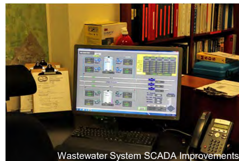
Wastewater System SCADA Improvements
