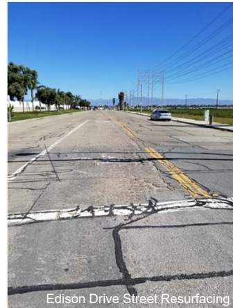
Edison Drive Street Resurfacing
