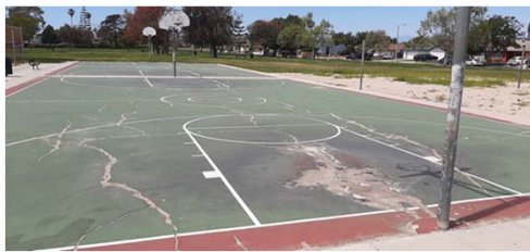
Basketball Court Resurfacing
