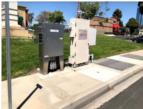
Lift Station No. 24 Improvements
