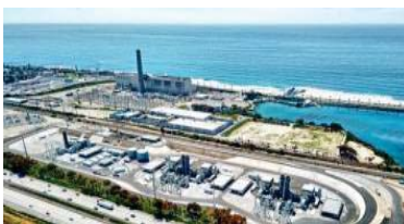
Encina Power Plant - 2017
