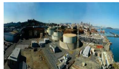
Potrero Generating Station - 2011
