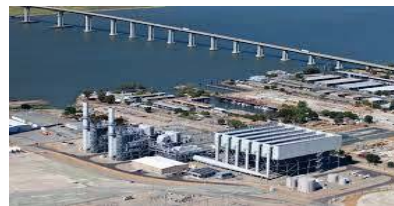
Gateway Generating Station - 2013
