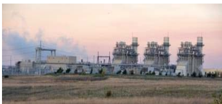
Delta Energy Center - 2016
