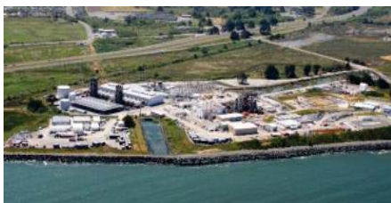
Humboldt Bay Power Plant - 2010
