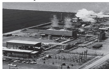
Daggett SCE Coal Water Gasification Plant - 1998
