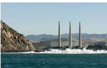
Morro Bay Power Plant - 2014
