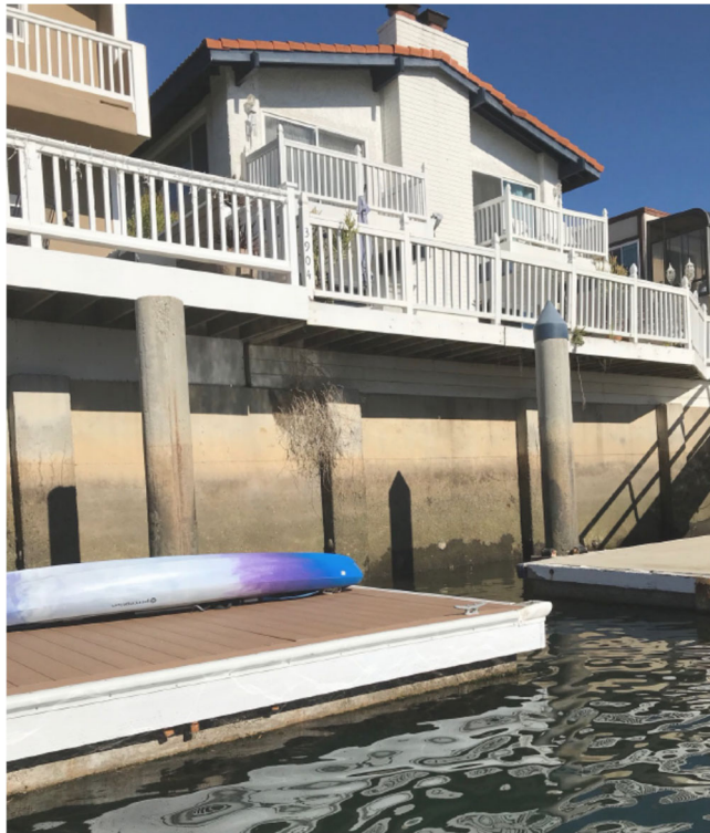
Figure 10 - Typical overhanging decks
