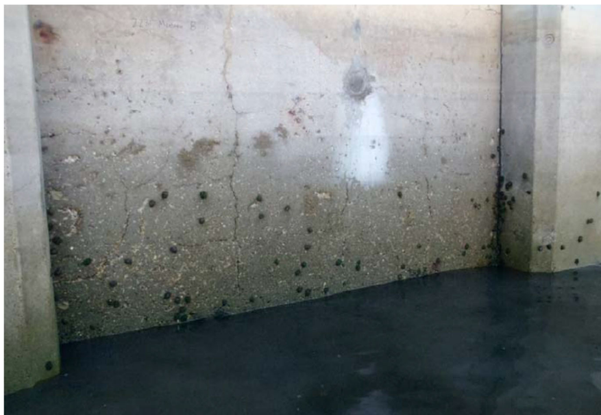
Figure 6 - Surface erosion and vertical cracking on a Boise wall panel [from TranSystems (2011)]
