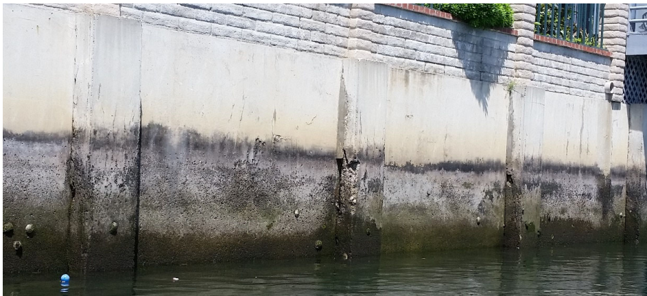
Figure 4 - Surface erosion/marine attack on Boise wall panels with cracking and spalling at pilasters
