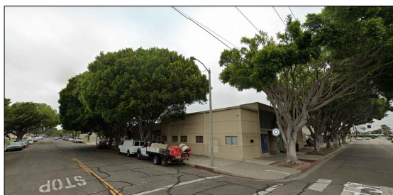
VIEW LOOKING NORTHEAST FROM INTERSECTION OF S. B ST. AND W. 2ND ST. 05
