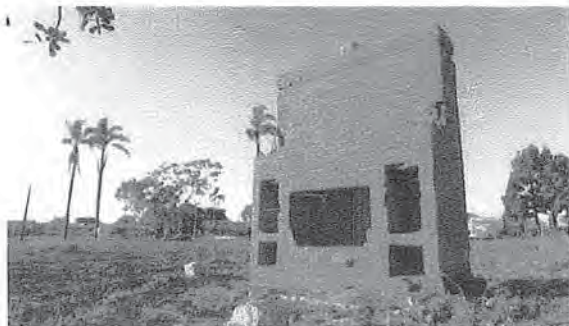
The Colonial House is a 'missed opportunity.' Once one of the most culturally significant structures in Oxnard, it was demolished in 1988. 20 years later, only a chimney stands testament to the developments planned for this site that never materialized.
