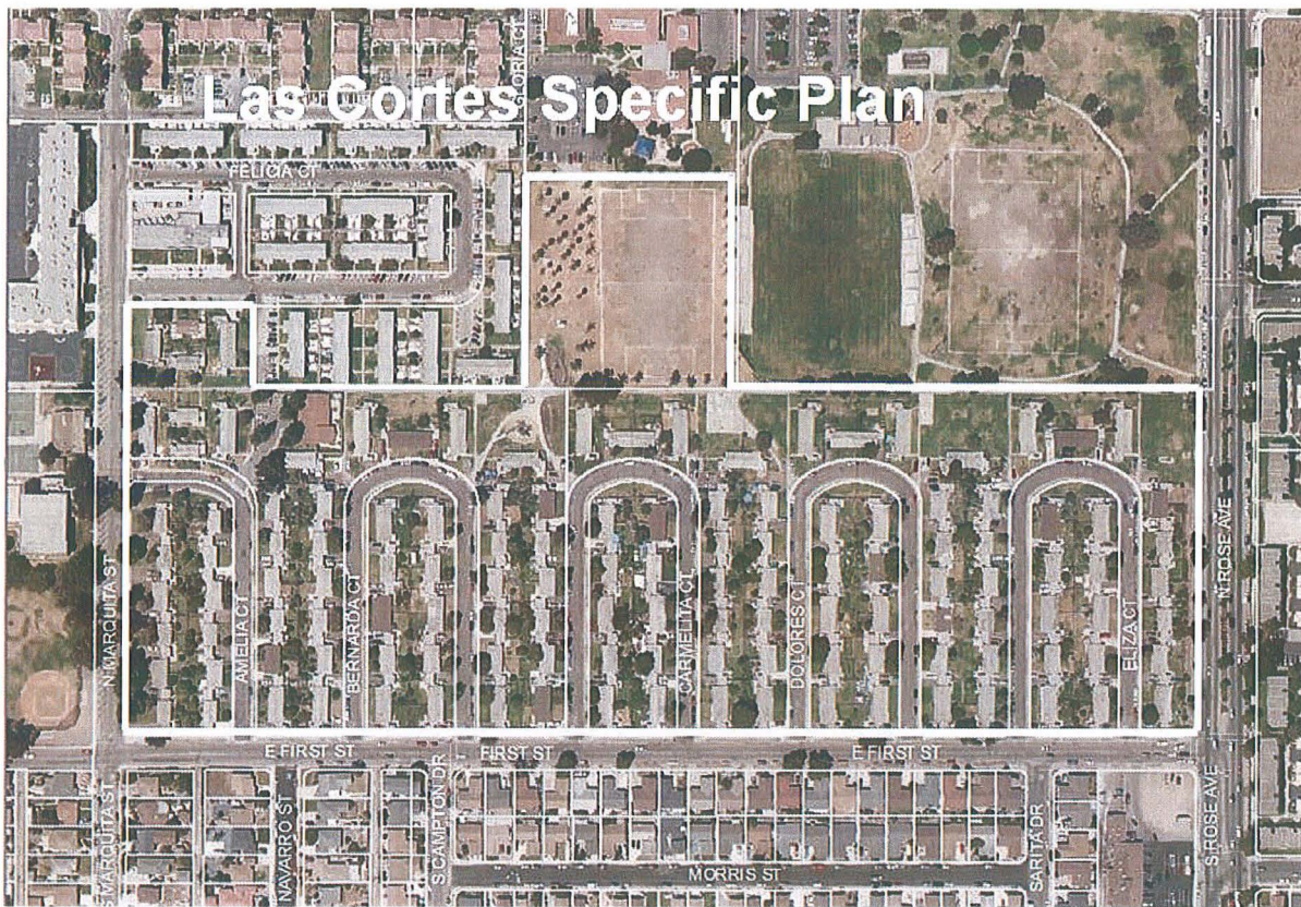
Figure 2: Existing (some demolition has occurred as of October, 2014) Development
