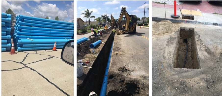
Installation of new PVC water main and PE services
