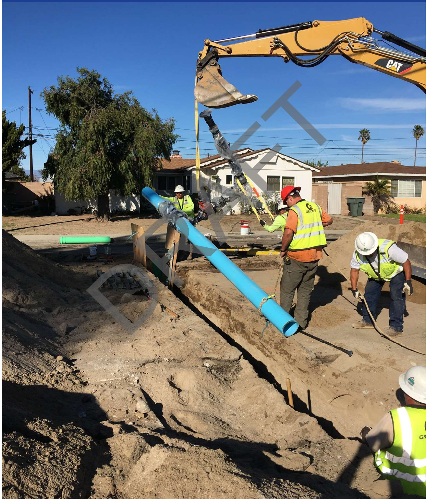
Cast Iron Pipe Replacement
