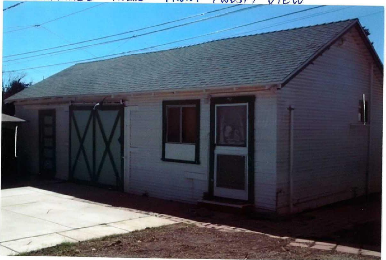
CARRIAGE HOUSE FRONT (WEST) VIEW
