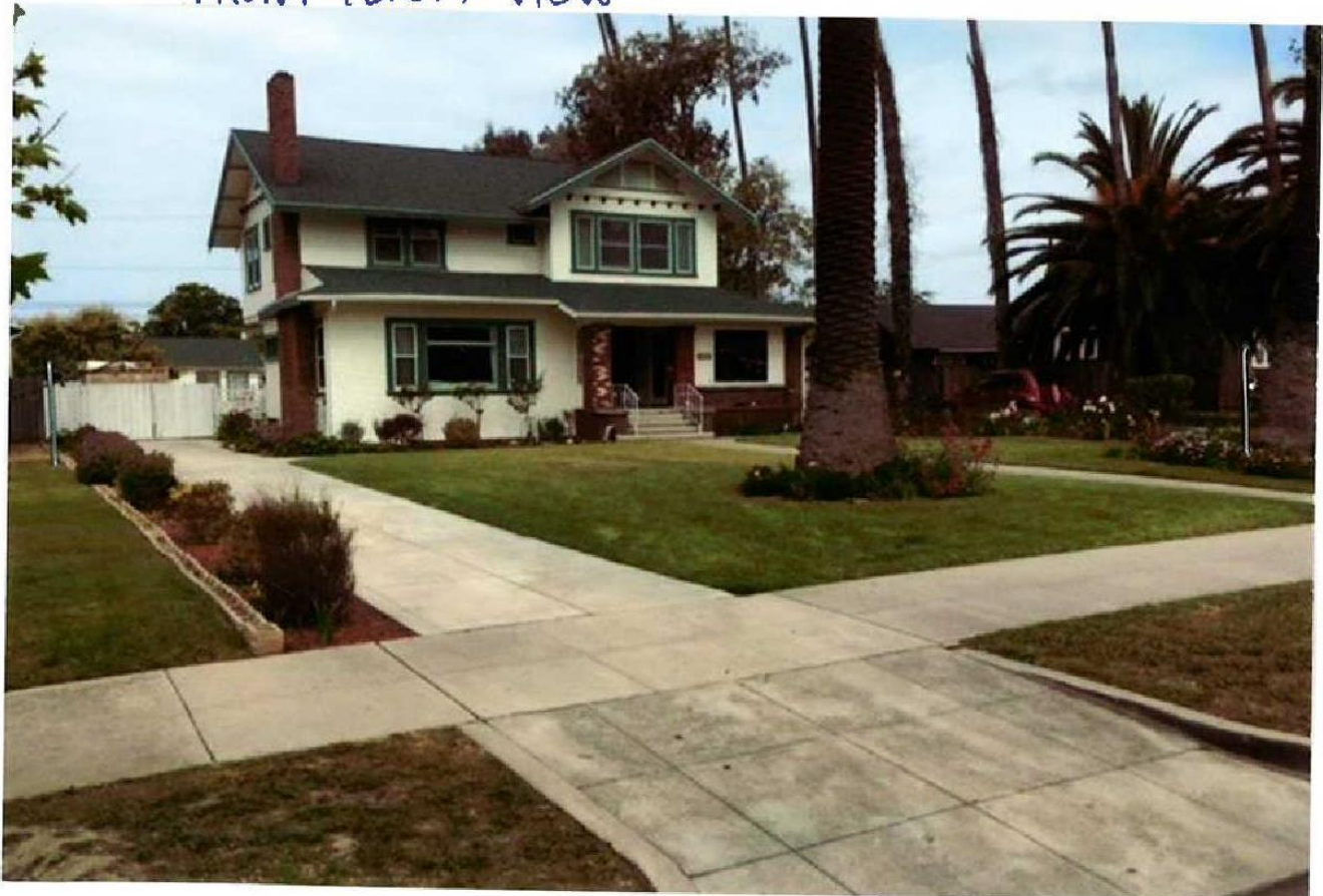
FRONT (EAST) VIEW
