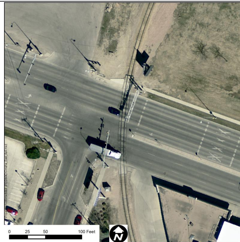
Omaha Avenue (East) (190267M)
