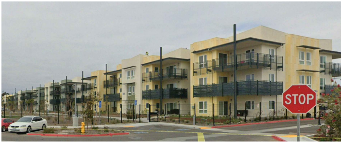
2. Surrounding Context - E. Wooley Rd. (looking east)
