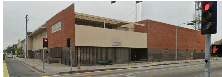
4. Site adjacent - south of site - S. C Street & 9th Street looking southeast)
