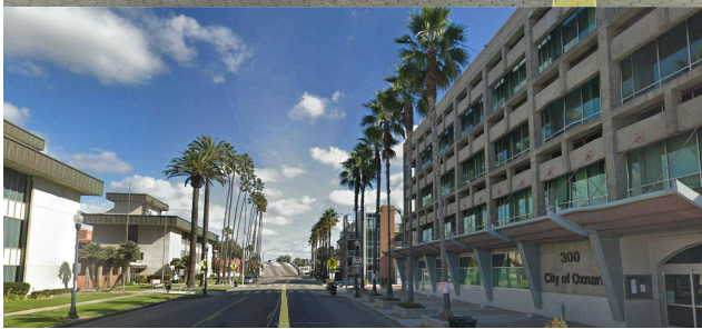
1. Surrounding Context - 3rd Street City Hall (looking east)
