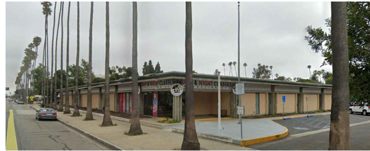
5. Existing Site - S. C Street looking south)
