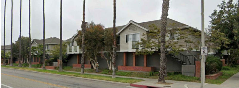
1. Site adjacent - east of site - S. C Street & 8th St. (looking east)
