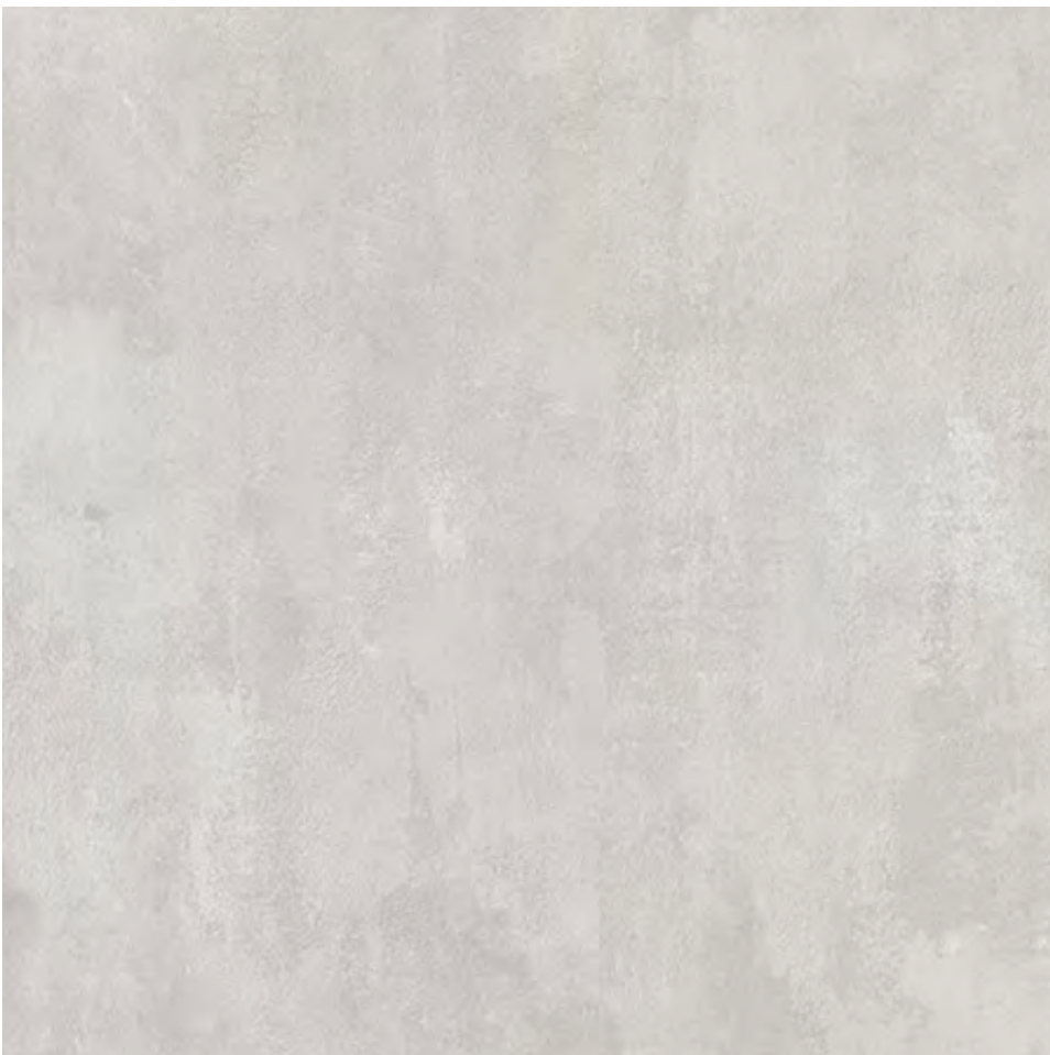
SMOOTH STUCCO TO BE PAINTED
