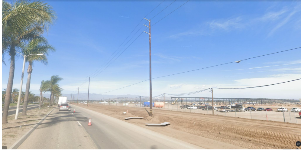
Current power line location (adjoining N/B Rice Ave. adjacent to Sakioka Farms)
