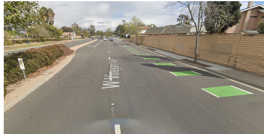
Vineyard Avenue – After (Buffered bike lanes, green paint at conflicts, bike detection)
