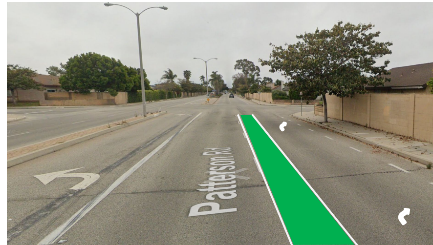
Patterson Road – Near Oarfish (Separated & widened bike lanes, improved Intersection channelization)
