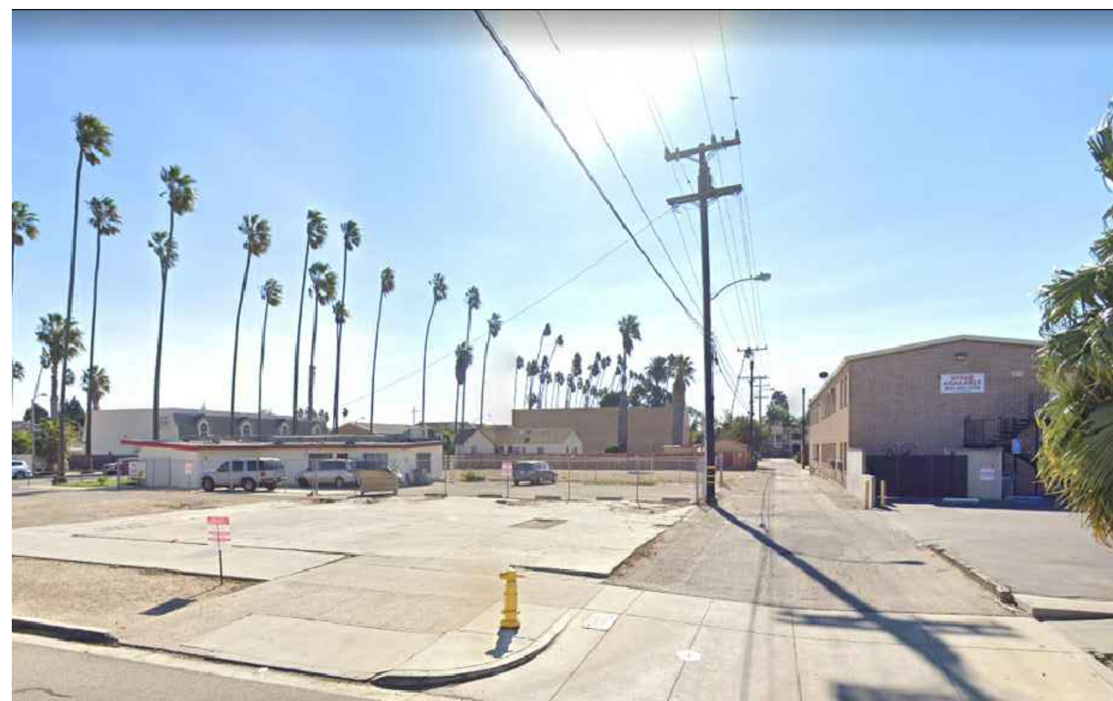
SOUTH VIEW AT ALLEY ③
