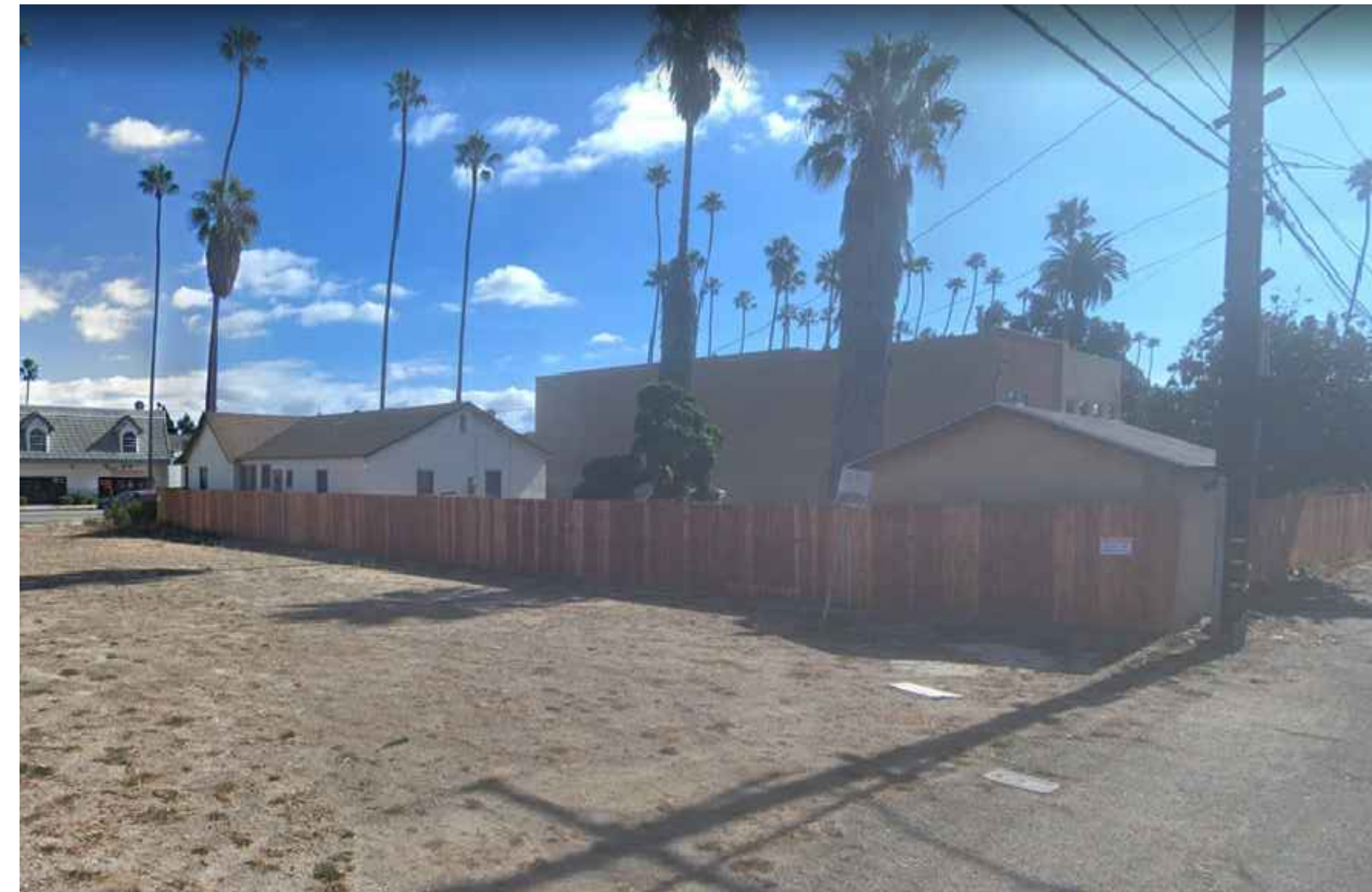
SOUTHEAST - ALLEY AT LOT ②
