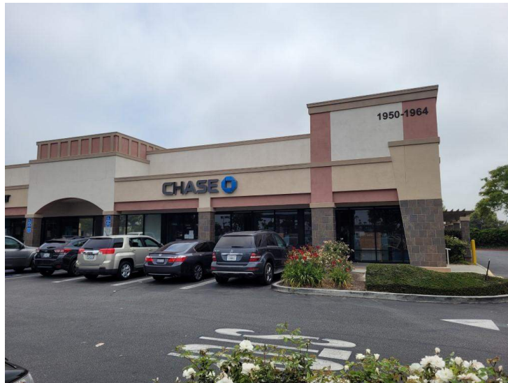
EXISTING SHOPPING CENTER LOOKING EAST FRONT ELEVATION & PARKING
