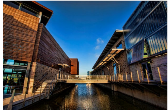
Figure 5 – Advanced Water Purification Facility, Oxnard
