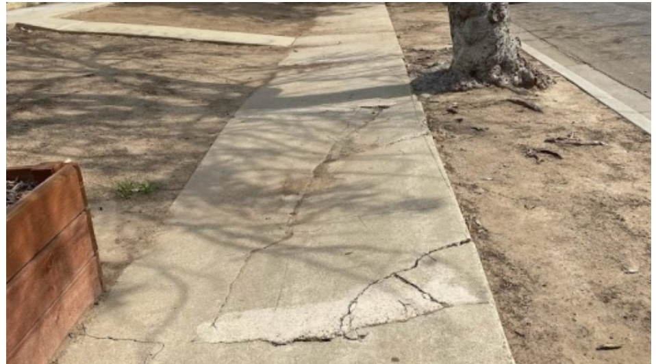
Citywide Sidewalk Repairs
