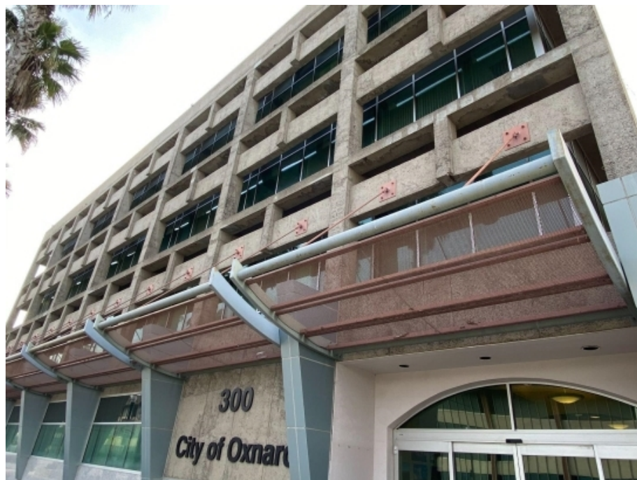
City Hall and Annex Exterior Improvements
