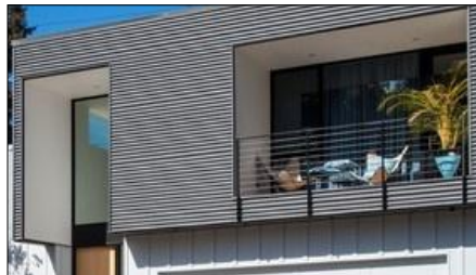
CONTRAST BETWEEN CORRUGATED METAL AND RECESSED PLAIN SURFACES
