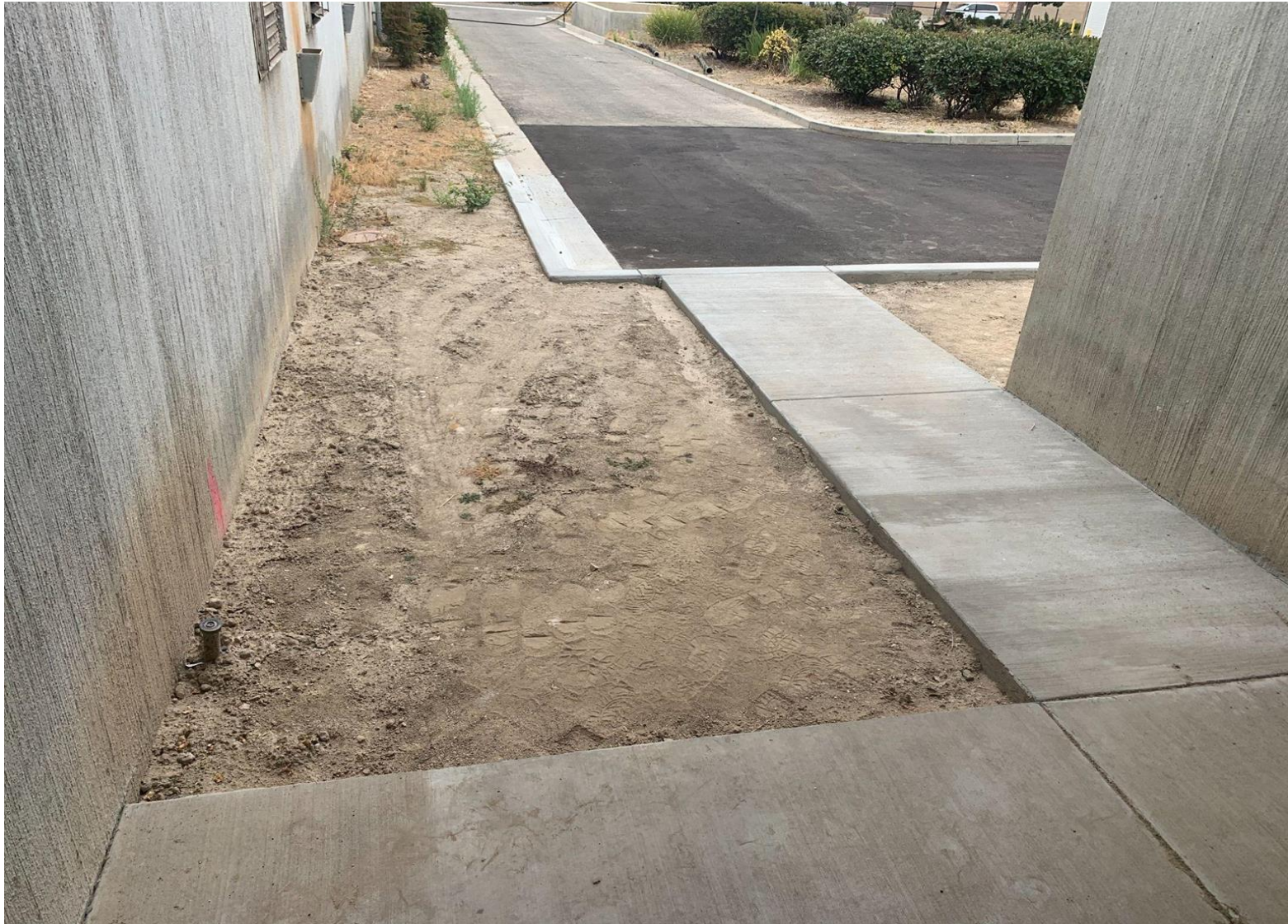
Completed repair of Tank Drainage at the OWTP
