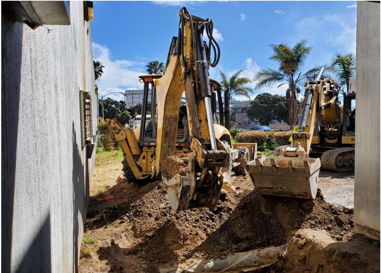
Urgent repair of Tank Drainage at the OWTP
