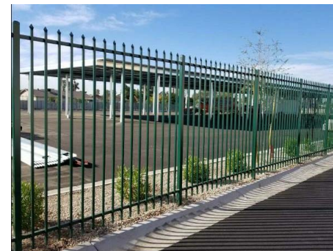
⑤ ANTI-CUT / ANTI CLIMB FENCING PHOTO 1/4" = 1'-0"
