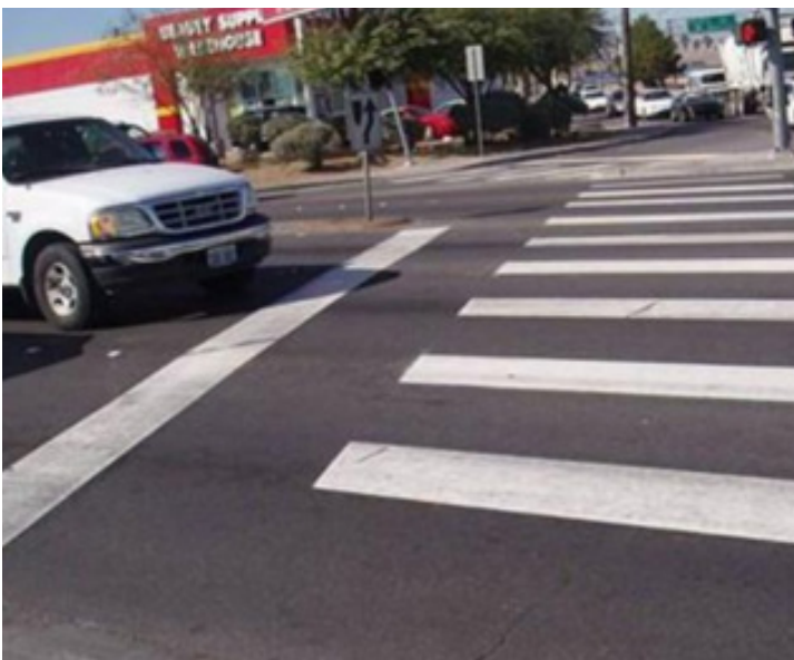
Advanced Stop Bar and High Visibility Crosswalks
