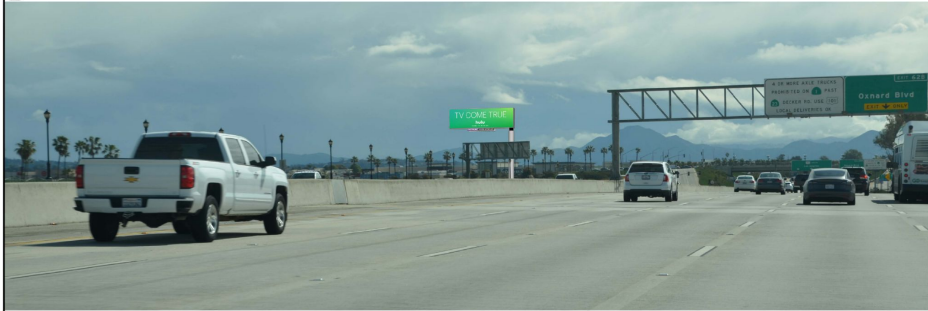
4 View From Southbound On U.S. 101
