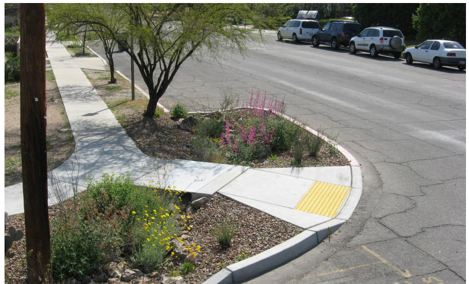
Example of a bulbout with landscaping for stormwater retention in Tucson, Arizona
