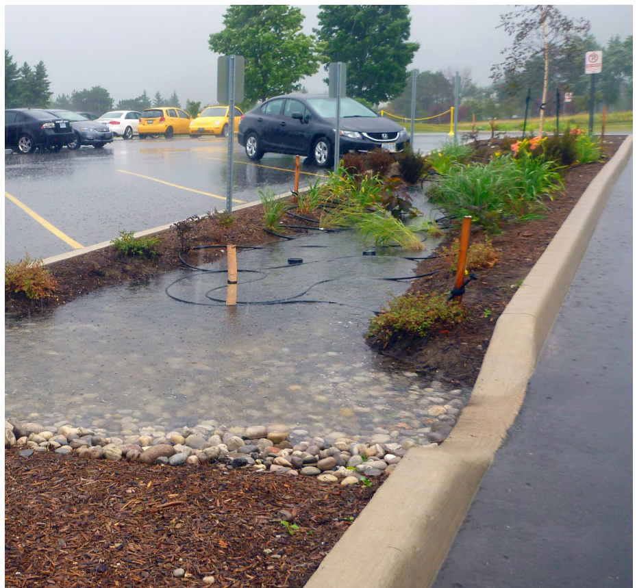
A bioswale with an inlet gathers stormwater that would have pooled in this parking lot. Source: Sustainable Technology Evaluation Program
