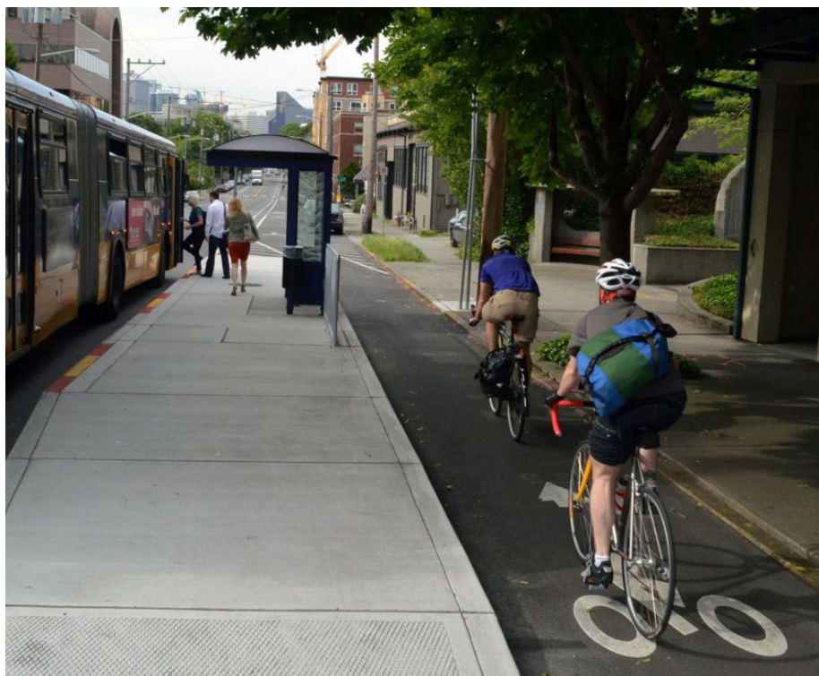
Side boarding island stops separate the boarding area from the sidewalk with a bike lane. Source: NACTO.
