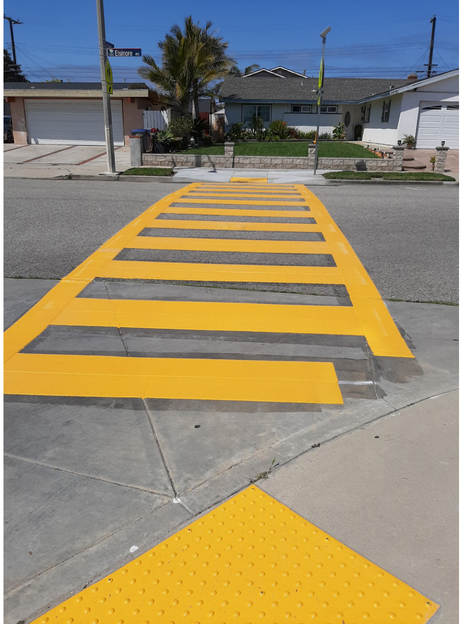
Upgraded curb ramps can alert visually impaired pedestrians of a pedestrian crossing. Source: City of Oxnard.
