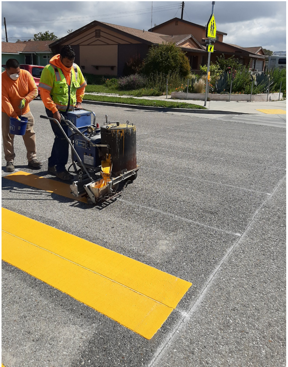
High-visibility crosswalks can be installed as part of road resurfacing projects. Source: City of Oxnard
