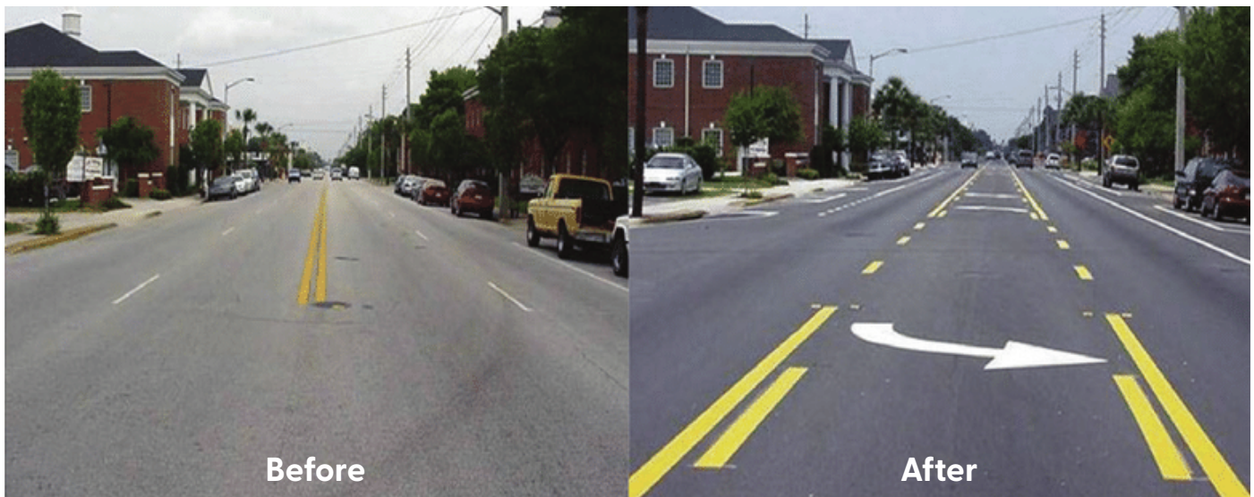
Road diets reallocate vehicle lane space to bicycle and pedestrian facilities. Source: NACTO.
