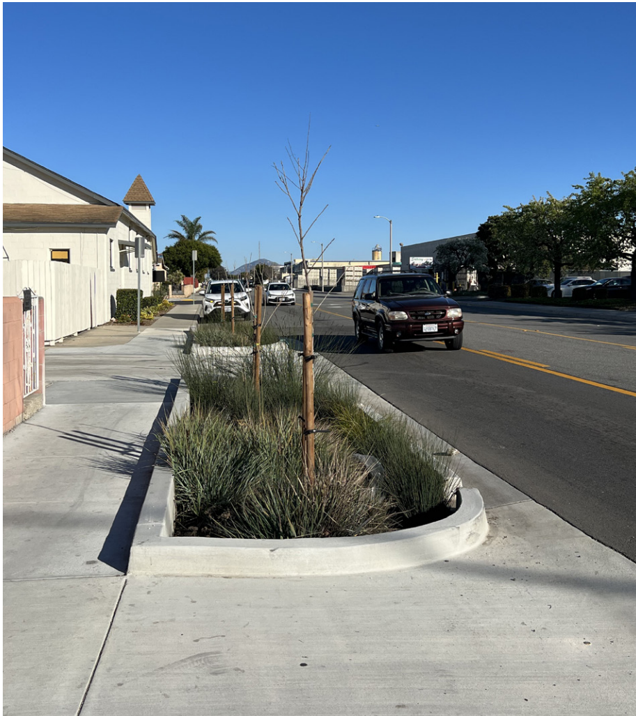
A planted median and bulbout visually narrow the travel lane to slow vehicle speeds. Source: City of Oxnard
