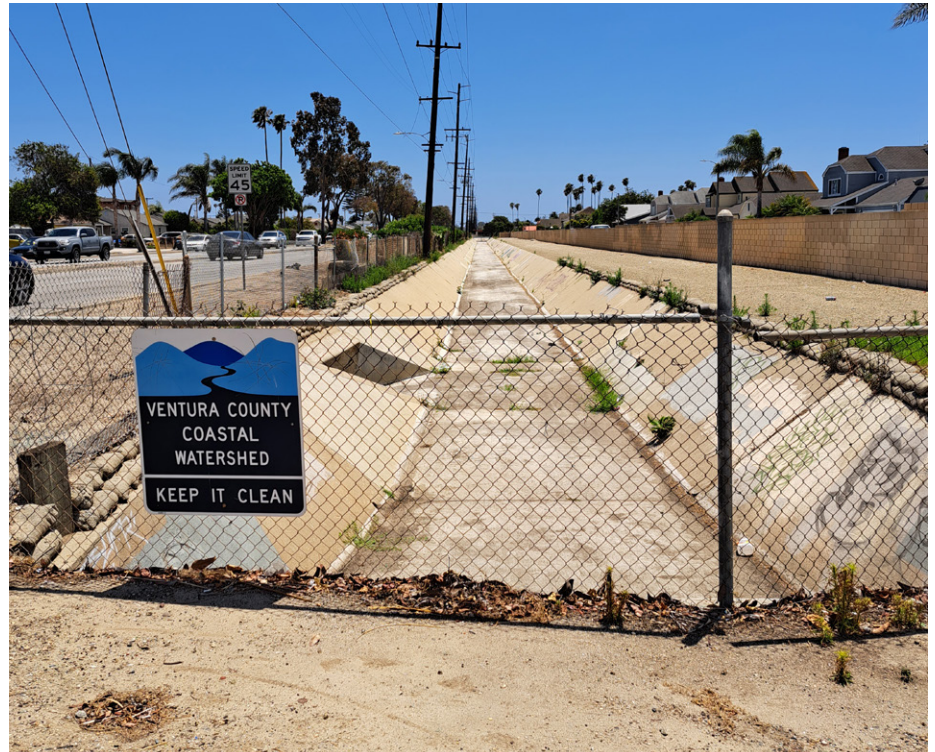
Existing flood channel along Wooley Road
