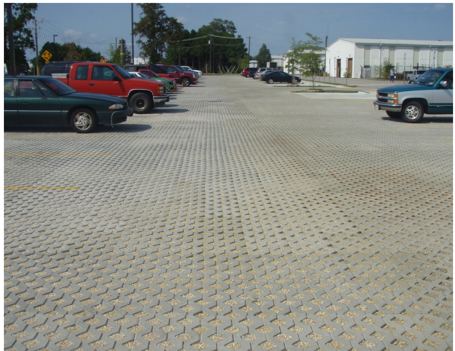
Parking lots can be an opportunity to incorporate permeable pavements. Source: US Army Corps of Engineers
