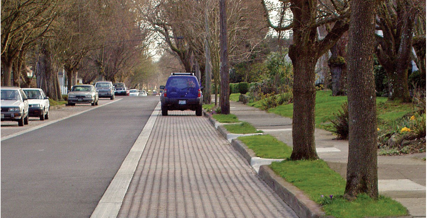
Parking lanes may be an opportunity to incorporate permeable pavement as they have less activity compared to the travel lane and receive the runoff draining from the crown of the roadway. Source: Portland Department of Transportation
