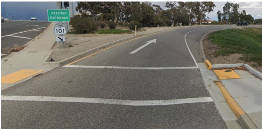
Existing upgraded curb ramps at freeway ramp along Vineyard Avenue
