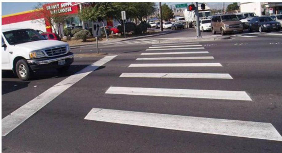
Advance stop bar and high-visibility crosswalk treatments at intersection Source: FHWA
