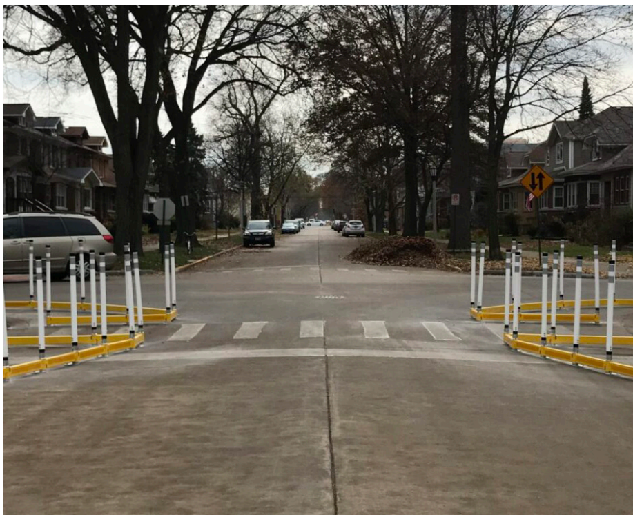
Curb extensions built with plastic posts can be a quick build option that also account for stormwater flow. Source: DeziLine
