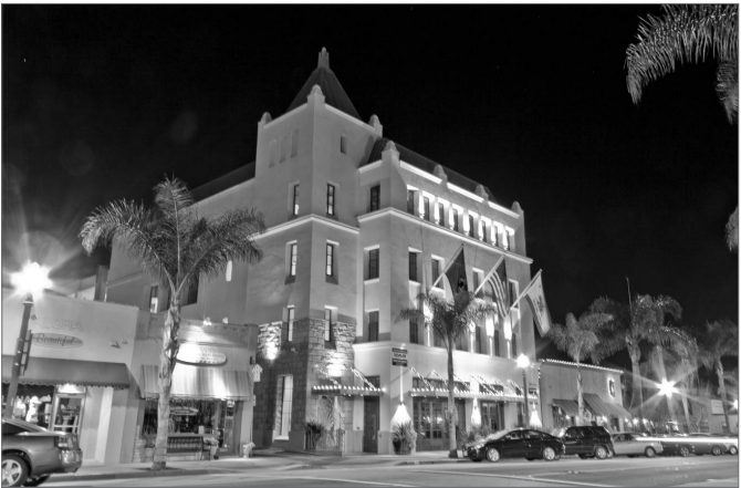
New downtown Ventura mixed-use infill building.
