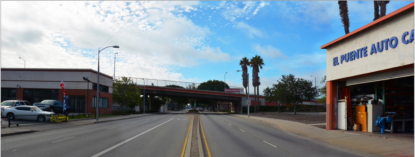
Existing Condition: The 3 rd St Bridge over crossing Oxnard Blvd provides a unique opportunity for gateway graphics and elements to alert and direct southbound travelers to Downtown.
