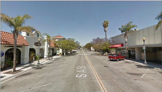
b Existing Condition (‘A’ St Downtown): Two travel lanes and angled parking have been restored to A Street south of 3rd, but more business activity and street beautification are needed.
