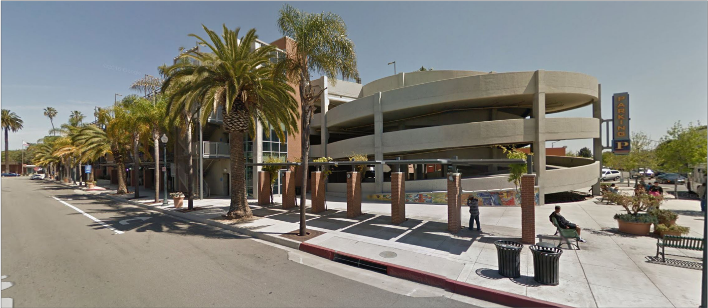
The Downtown Oxnard Parking Structure, at the corner of 4th and B Streets, provides 440 spaces just north of Downtown.
