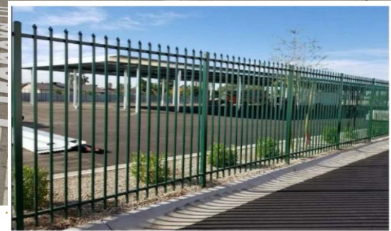
ANTI-CUT / ANTI-CLIMB FENCING PHOTO 1/4" = 1'-0"
