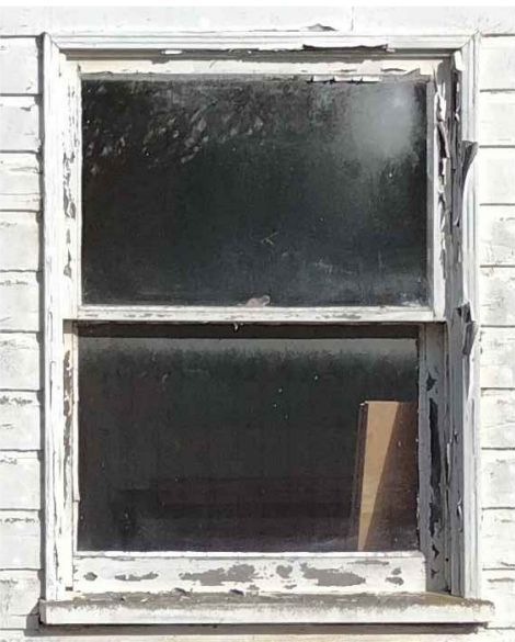
EXISTING WINDOWS: TO BE REMOVED & REPLACED
