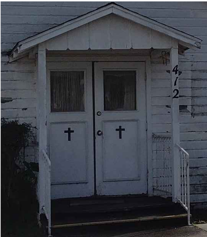
EXISTING ENTRY DOOR: TO BE REMOVED
