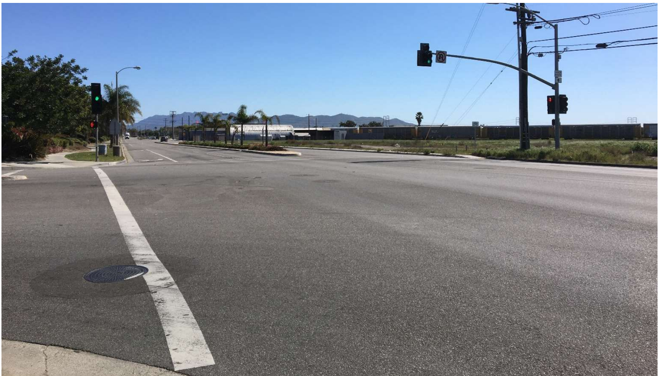
D - VIEW OF INTERSECTION AT HUENEME RD, LOOKING EAST
