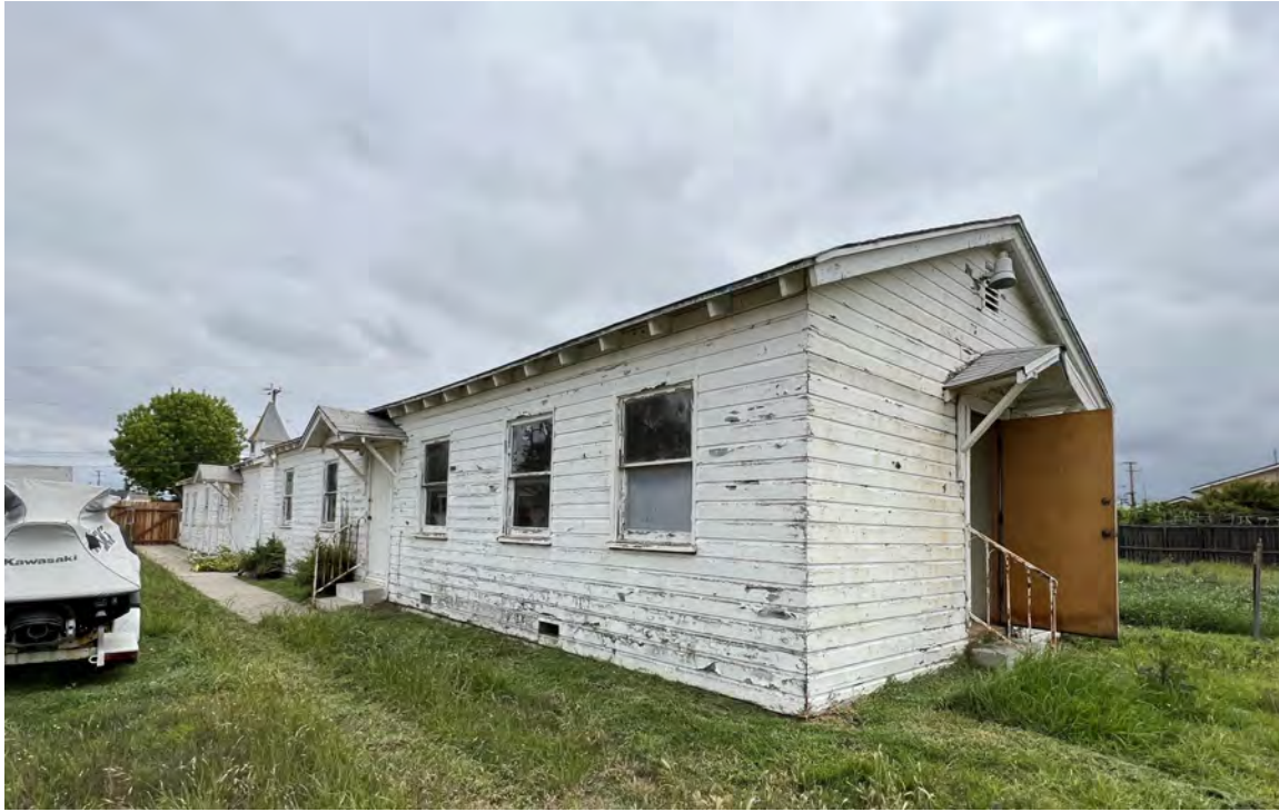
Photo 8: West elevation, view looking northeast. (GPA Consulting, June 2023).
