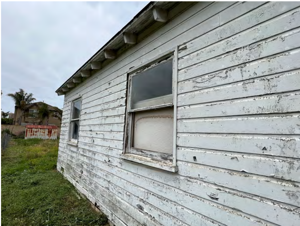
Photo 5: East elevation, view looking southwest. (GPA Consulting, June 2023).
