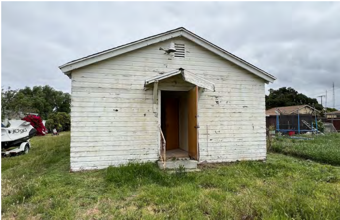
Photo 9: South elevation, view looking north. (GPA Consulting, June 2023).
