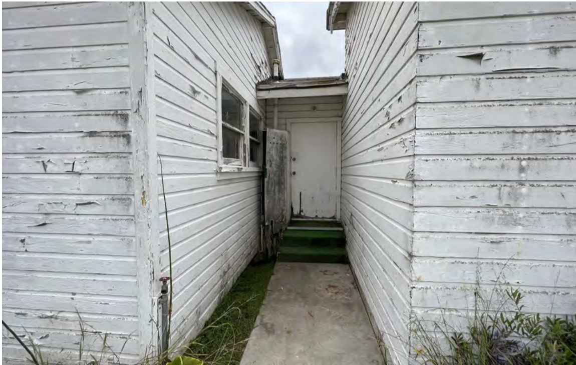
Photo 7: West elevation, view looking northeast. (GPA Consulting, June 2023).
