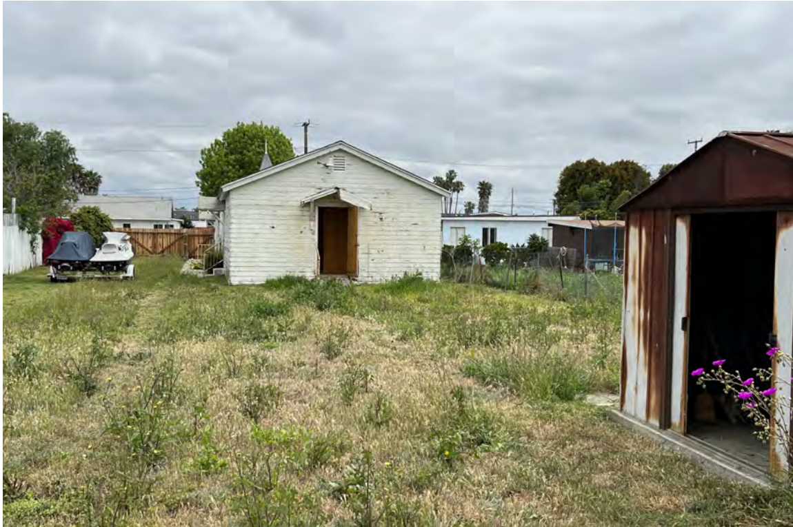
Photo 10: South elevation, view looking north. (GPA Consulting, June 2023).
