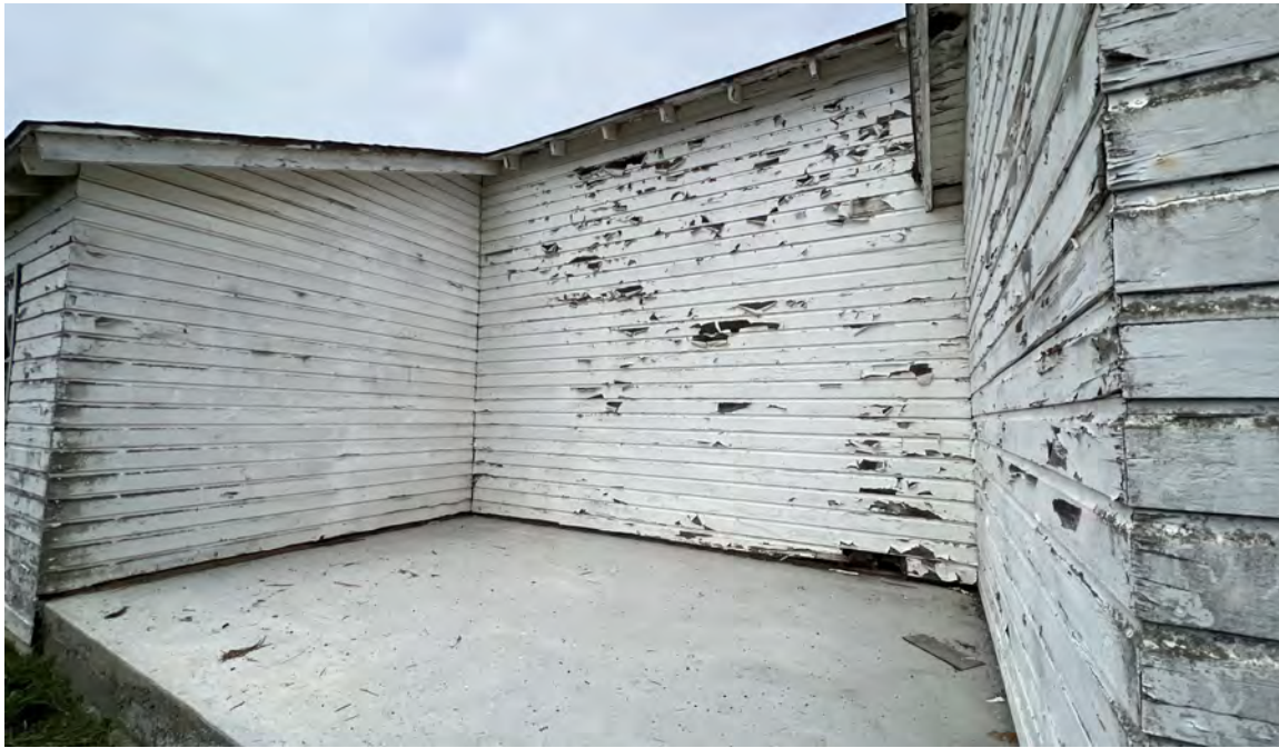
Photo 4: East elevation, view looking southwest. (GPA Consulting, June 2023).
