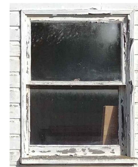
EXISTING WINDOWS: TO BE REMOVED & REPLACED
