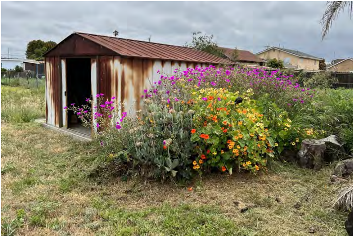
Photo 11: Prefabricated shed, view looking southeast. (GPA Consulting, June 2023).
